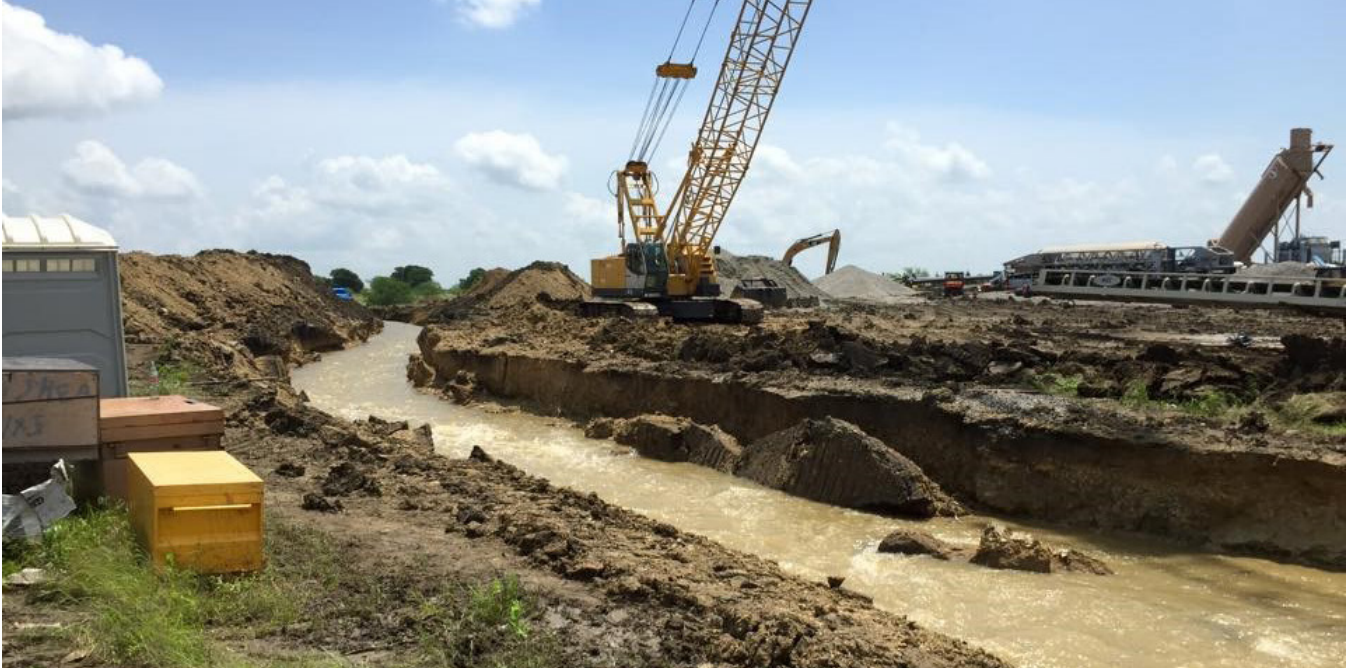
Figure 18: Bypass Channel Constructed around Cofferdam to Prevent Overtopping of Erodible Structure
