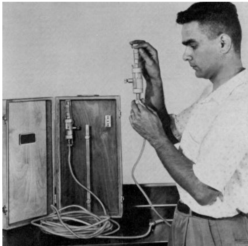
Figure 4-20. Autocollimating Tilt Measurement System
