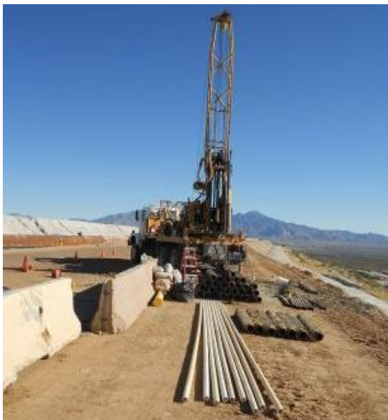
Photo 5: Auger Drill Rig
