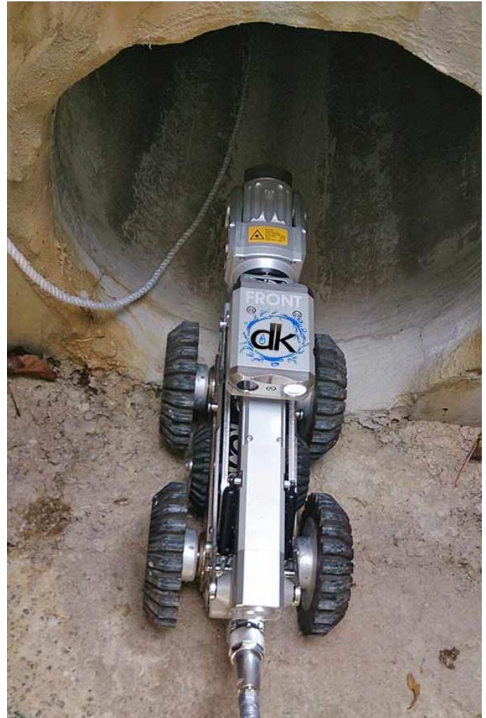
Figure 2. CCTV Camera on a Pipe-Crawler Being Inserted into a Conduit (courtesy Drains Kleen).
