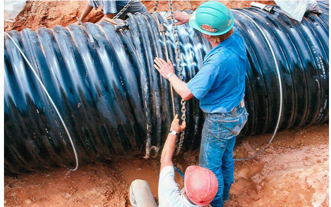
Figure 1. A CMP Conduit Being Installed [1].
