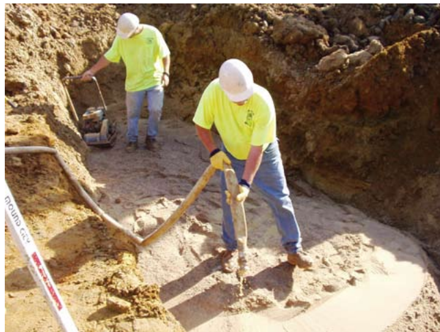
(d) Adding water to sand in filter diaphragm excavated below grade of principal spillway conduit prior to compacting
