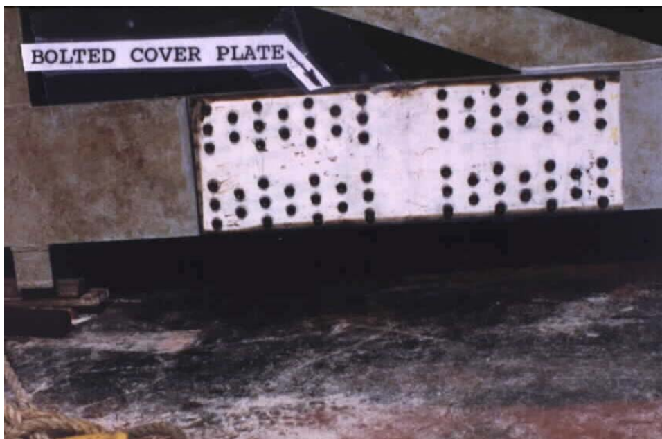
Figure 8-15. Bolted repair splice for the girder shown in Figure 8-13
