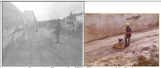
Construction Photographs of Filter Placement around the Conduit
