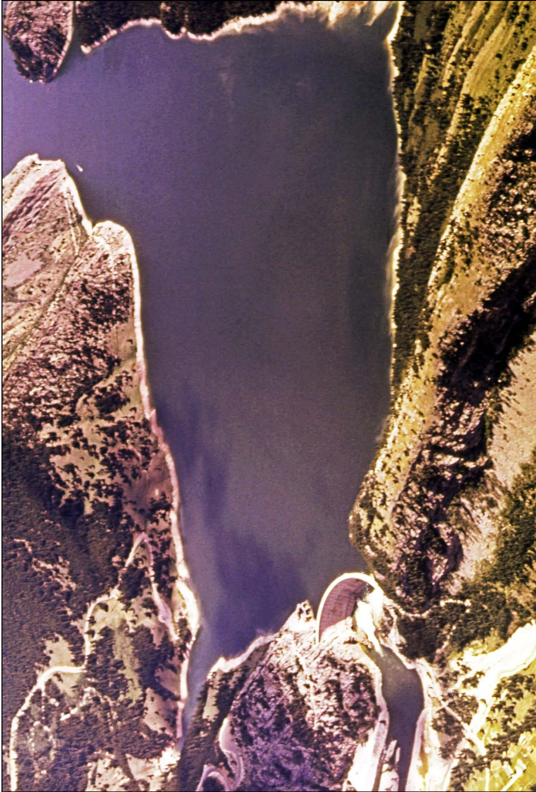
Photo 1.2.2.1-1. Gibson Dam (near Augusta, Montana).
