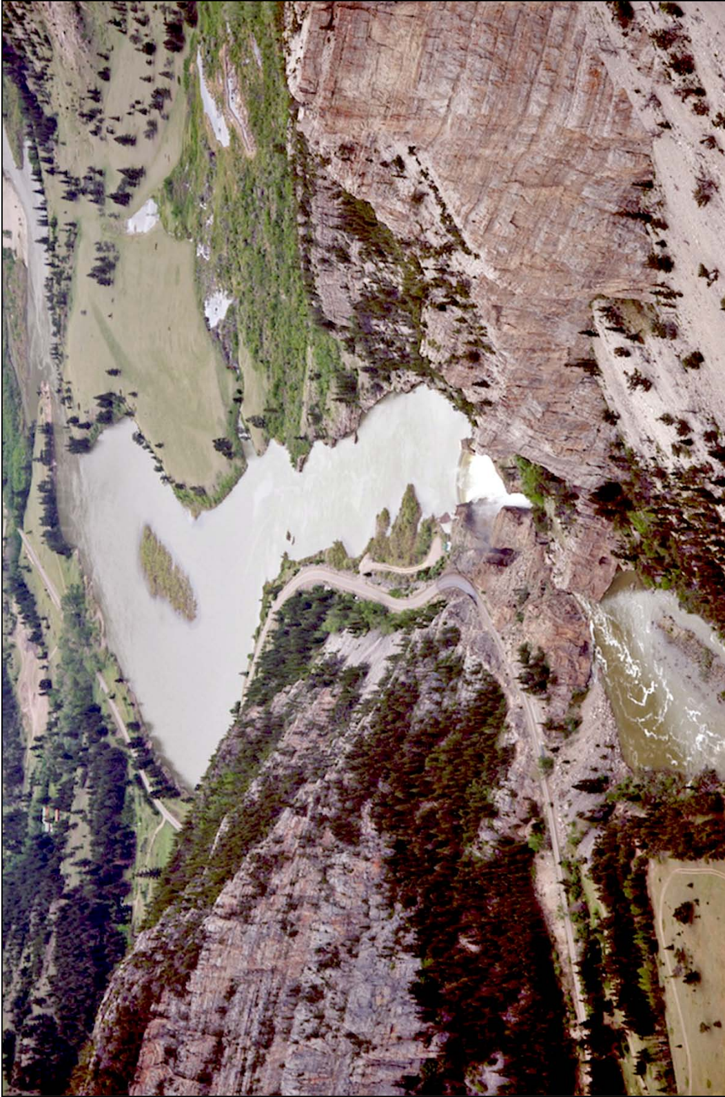
Photo 1.2.1.2-1. Sun River Diversion Dam (near Great Falls, Montana).
