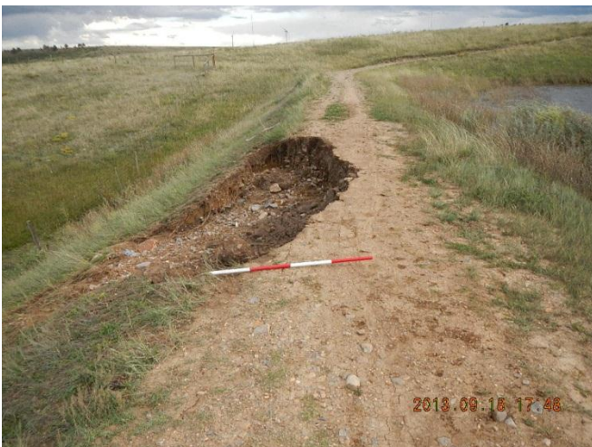
Photo 3. Slope failure on downstream slope
