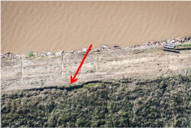
Photo 1. Severe longitudinal cracks in downstream slope
