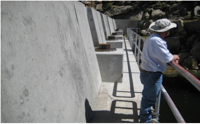
Figure 19 – Photo of Anchors Installed through Right Abutment Arch Section.
