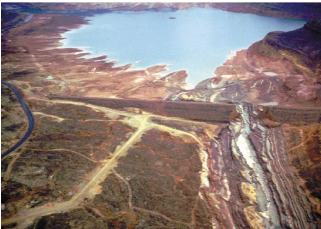
Figure 15 - Quail Creek Dike
