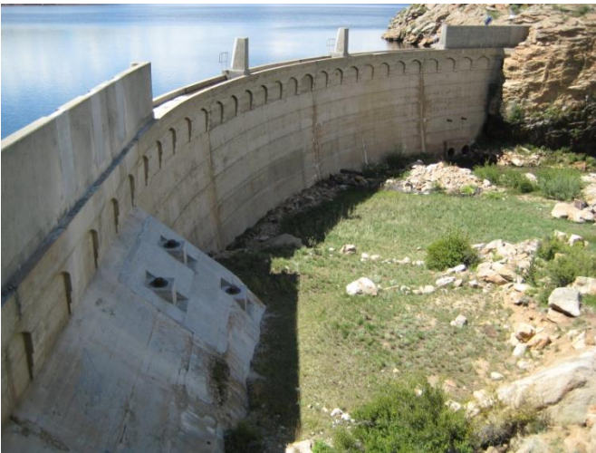
Figure 17 – Downstream Face of Tarryall Dam from the Right Abutment
