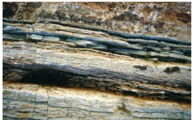
Figure 16 - Openings along Bedding Planes
