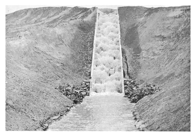
Baffle piers 18'' high and 18'' wide—18'' spaces. Row spacing, 6'0''. Chute 9' wide and 90' long—2 : 1 slope. Training walls 5' high. FIGURE 139.—Kopp Wasteway on the Main East Canal, Michaud Flats project, Idaho, discharging 25 c.f.s. (one-third capacity).
