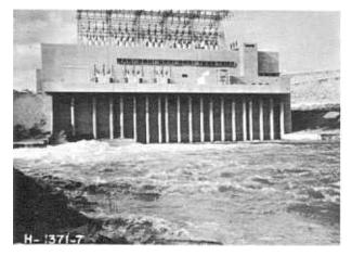
90-inch outlet works valves 100 percent open, discharging 4,500 c.f.s., approx. T.W. elevation 183.6. Turbine gates 72 percent open, 100 percent load.
