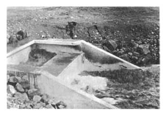
South Dam outlet works structure discharging 130 c.f.s. (80 percent of maximum).
