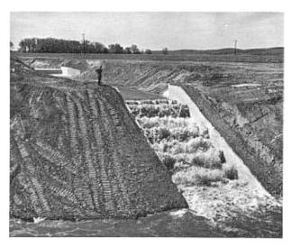
Baffled apron of Culbertson Canal Wasteway 3.3 discharging 75 c.f.s. Good performance. Design discharge 400 c.f.s.
