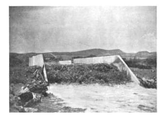
Estimated discharge 15 c.f.s. per foot width (half capacity).
