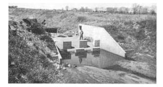
No flow through structure on Bostwick Courtland Canal, Drain A, Sta. 6+08, designed for 924 c.f.s.
