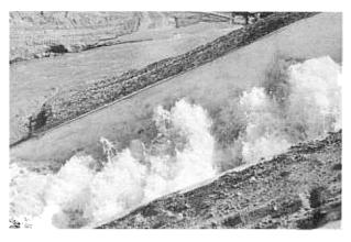
Same flow in midportion of chute. See right-hand photograph in Figure 134 for general view.
