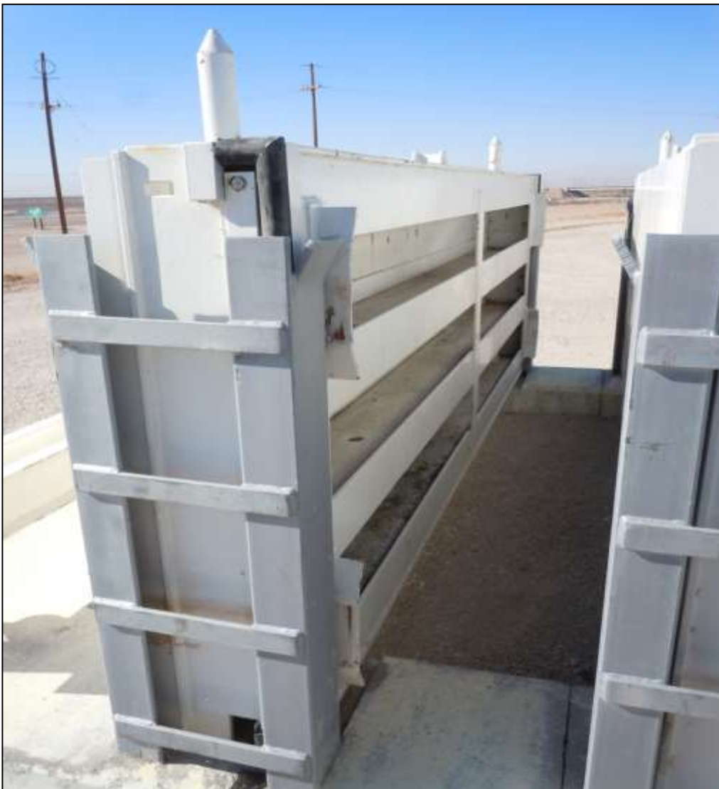
Figure 6.3.8-1. Stoplogs stored in the storage yard in vertical supports resembling the guides that are embedded in a concrete pad.
