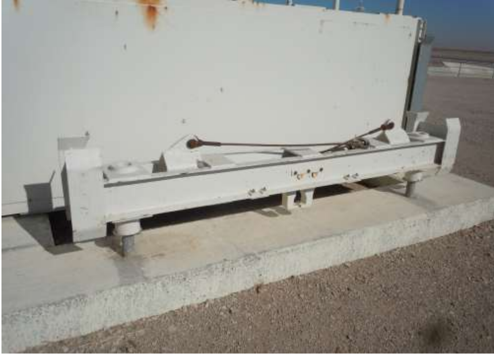
Figure 6.3.4-1. Lifting beam stored on concrete pad in yard. Note the stored stoplogs behind the lifting beam.
