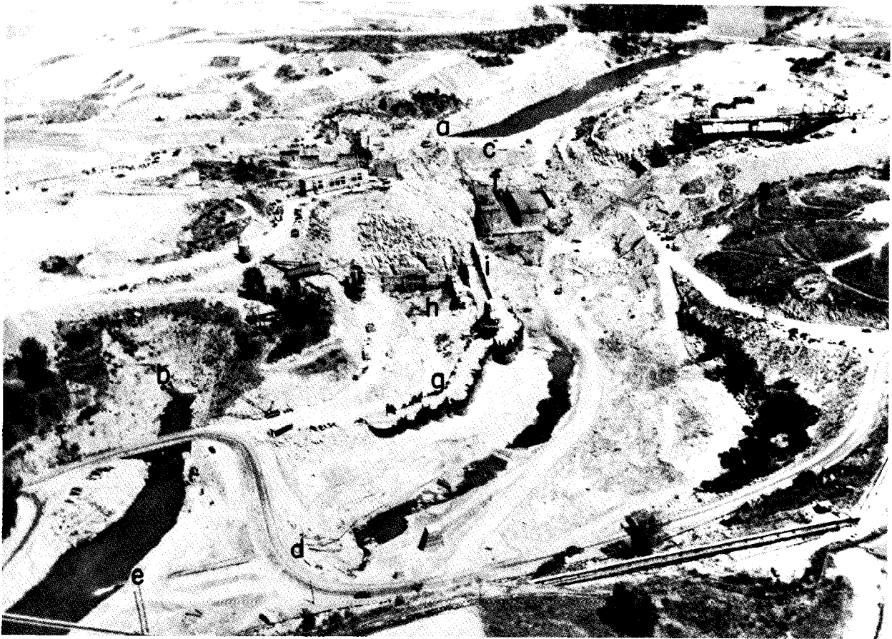
Figure 5-2. Diversion of the river during construction of Folsom Dam and Powerplant in California.-AR-16270.
