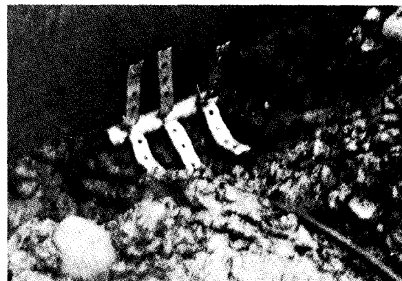
Figure 13-15. Resistance thermometer installed at upstream face of a dam.-3PXI 3/10/71-3
