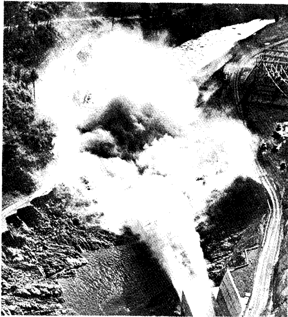
Figure 9-38. Deflector bucket in operation for the spillway at Hungry Horse Dam in Montana.-P447-105-5924
