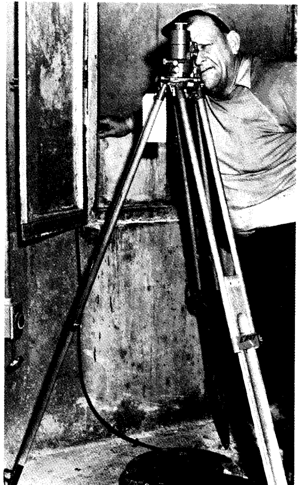
Figure 13-24. Foundation deformation well, optical plummet, and reference grid.—P459-6404221
