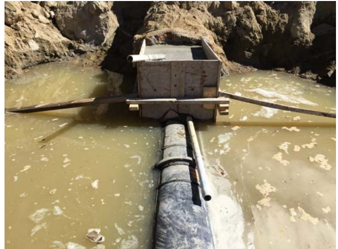
Figure 3. Cellular Grout Placement at Estler Lake Dam
