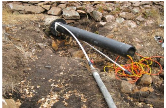
Photo 10: Grouting HDPE liner pipe. 3
