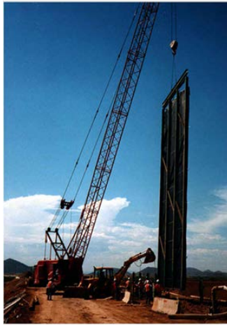
(a) Geomembrane panel installation and (b) top view of installed panels at Reach 11 Dikes.
