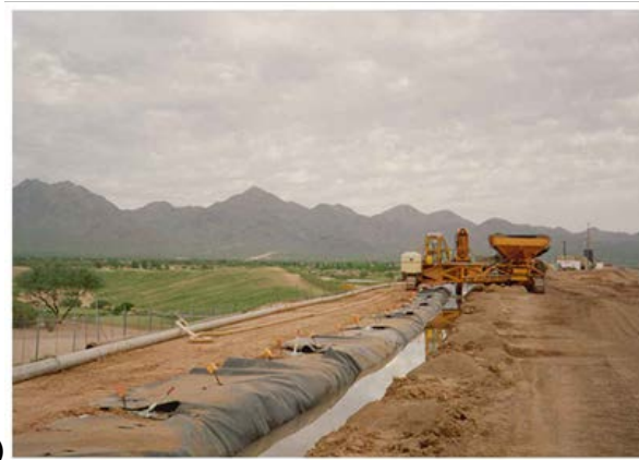
(a) Geomembrane panel installation and (b) top view of installed panels at Reach 11 Dikes.
