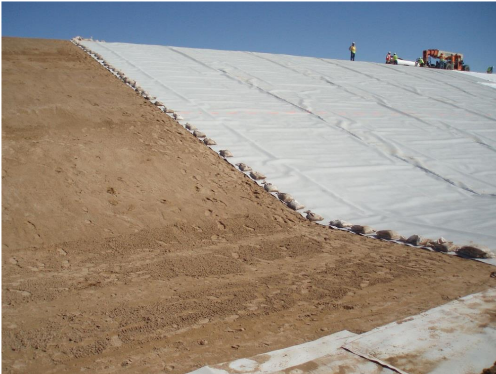
Figure 20.4.7.1-1. Temporary anchorage at leading edge of geomembrane with sandbags.
