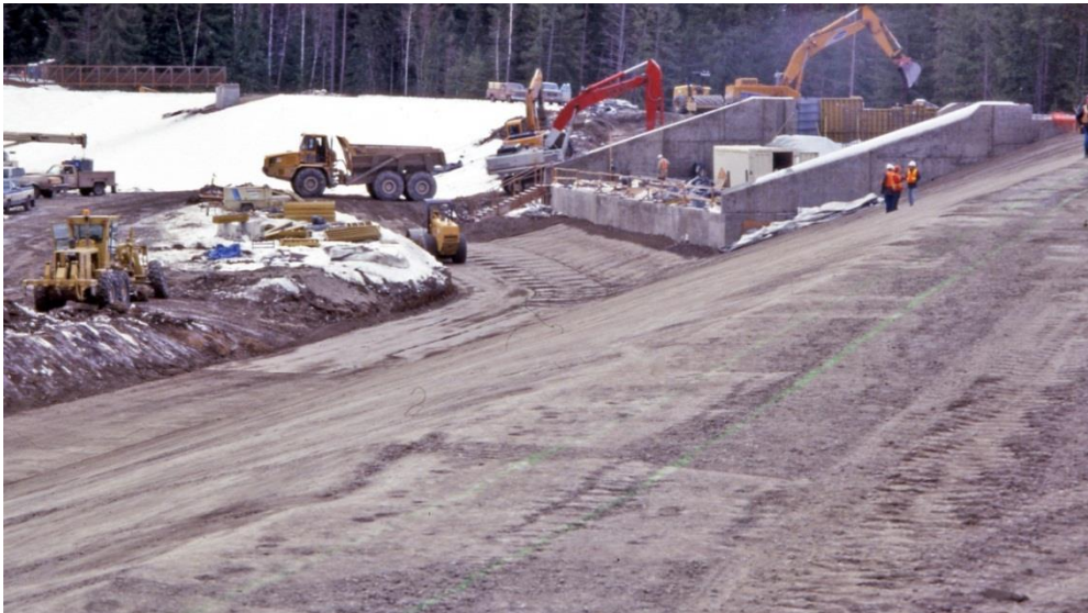
Figure 20.5.7.1-1. Subgrade preparation prior to geomembrane installation.
