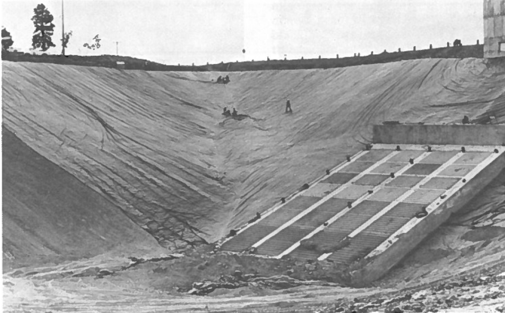
Figure 20.3.3.3-2. Six-man crew performing seaming operations near the Mt. Elbert inlet/outlet dike.
