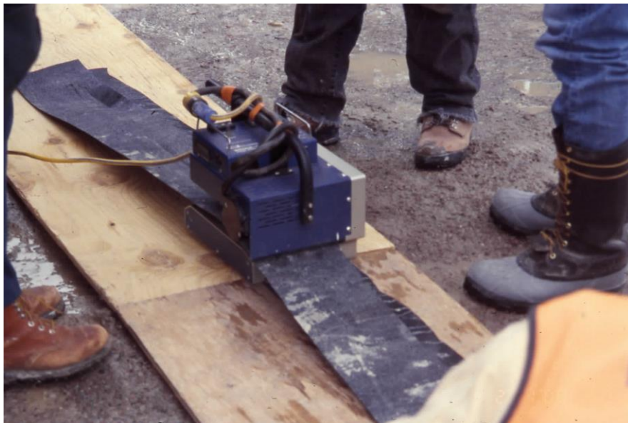
Figure 20.5.8.3-1. Trial seam performed on suitable, clean surface.
