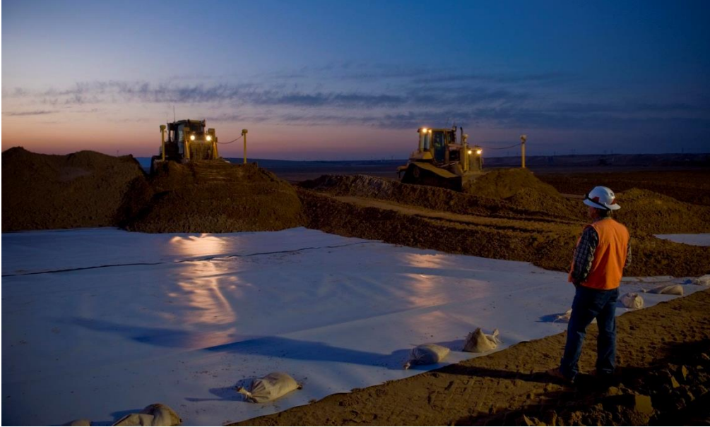
Figure 20.5.13.2-1. Placement of protective cover over a geomembrane.
