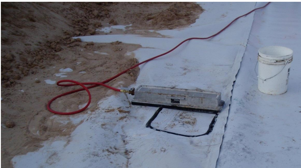
Figure 20.5.10.1-2. Vacuum testing of an extrusion welded patch.
