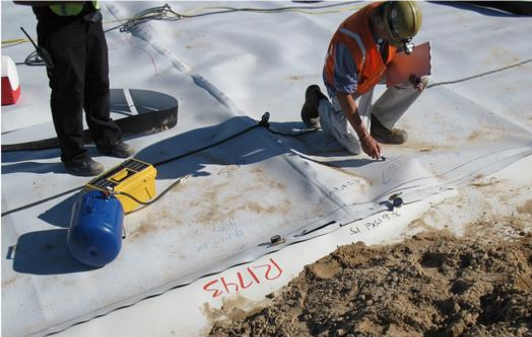
Figure 20.5.10.1-1. Air pressure testing of a dual-wedge-welded seam.
