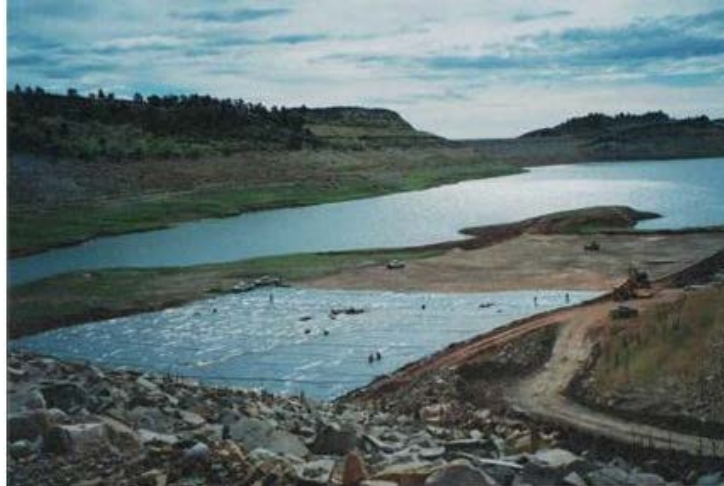
Figure 20.3.3.1-2. LLDPE geomembrane installation.
