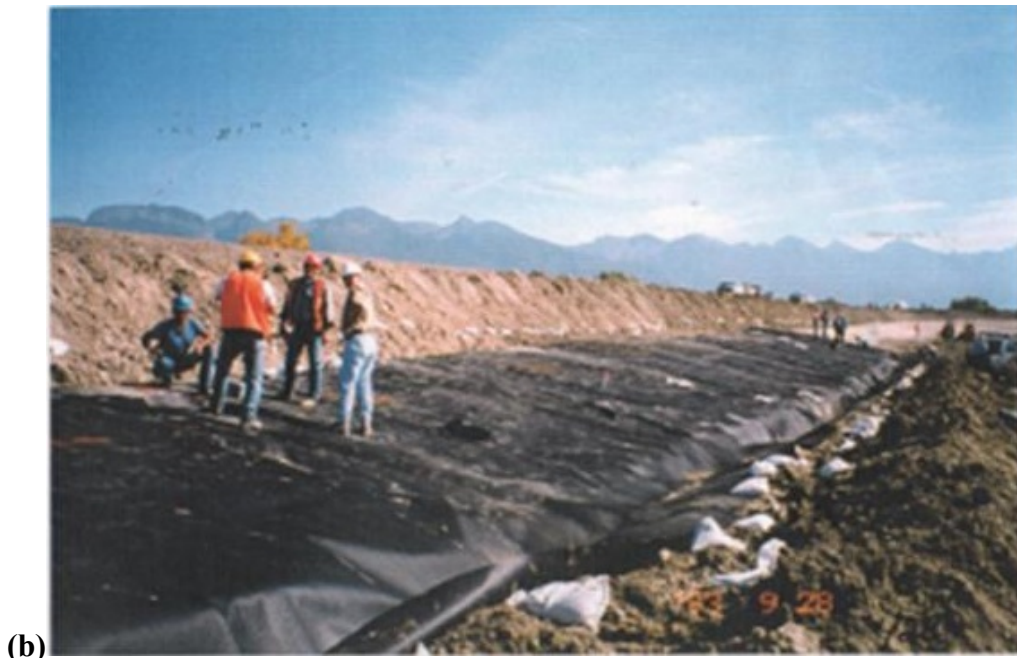
Figure 20.3.3.5-2. (a) Anchor trench excavation and (b) installation of geomembrane.
