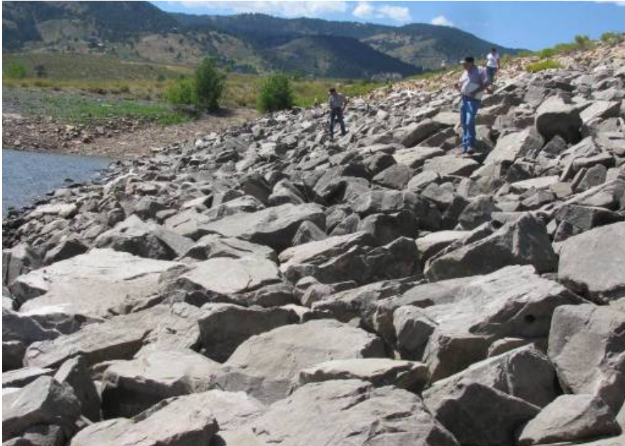
Figure 2.2.5.3.3-1. Riprap on upstream slope of Horsetooth Dam, Colorado.
