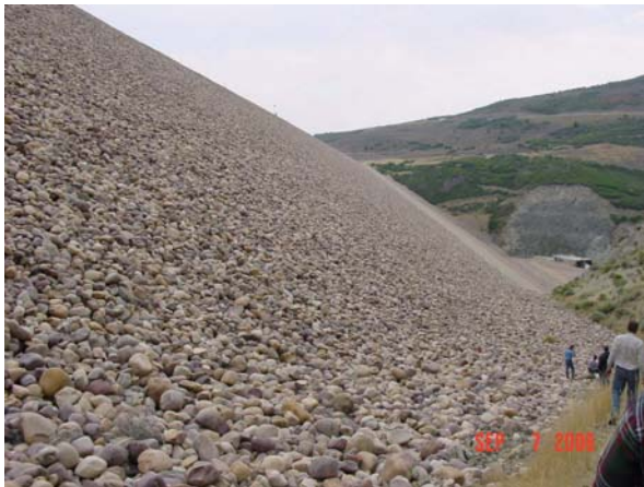
Figure 2.2.5.4-1. Cobble slope protection on downstream slope of Jordanelle Dam, Utah.
