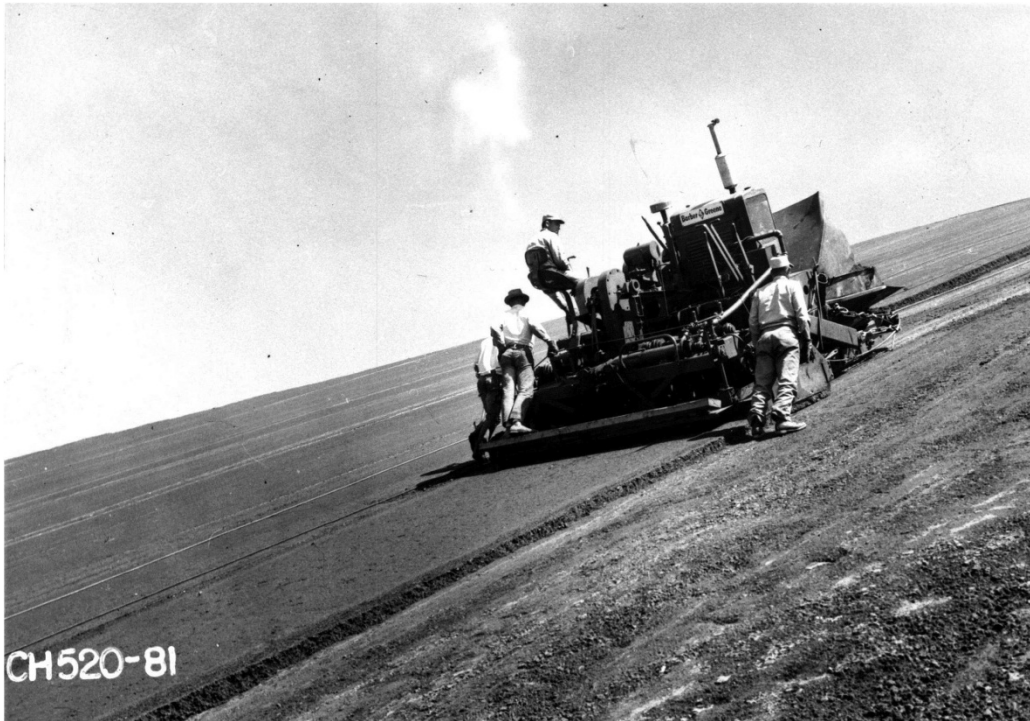
Figure 2.3.6.3-2. Placing asphaltic concrete on the upstream slope of Montgomery Dam, Colorado.
