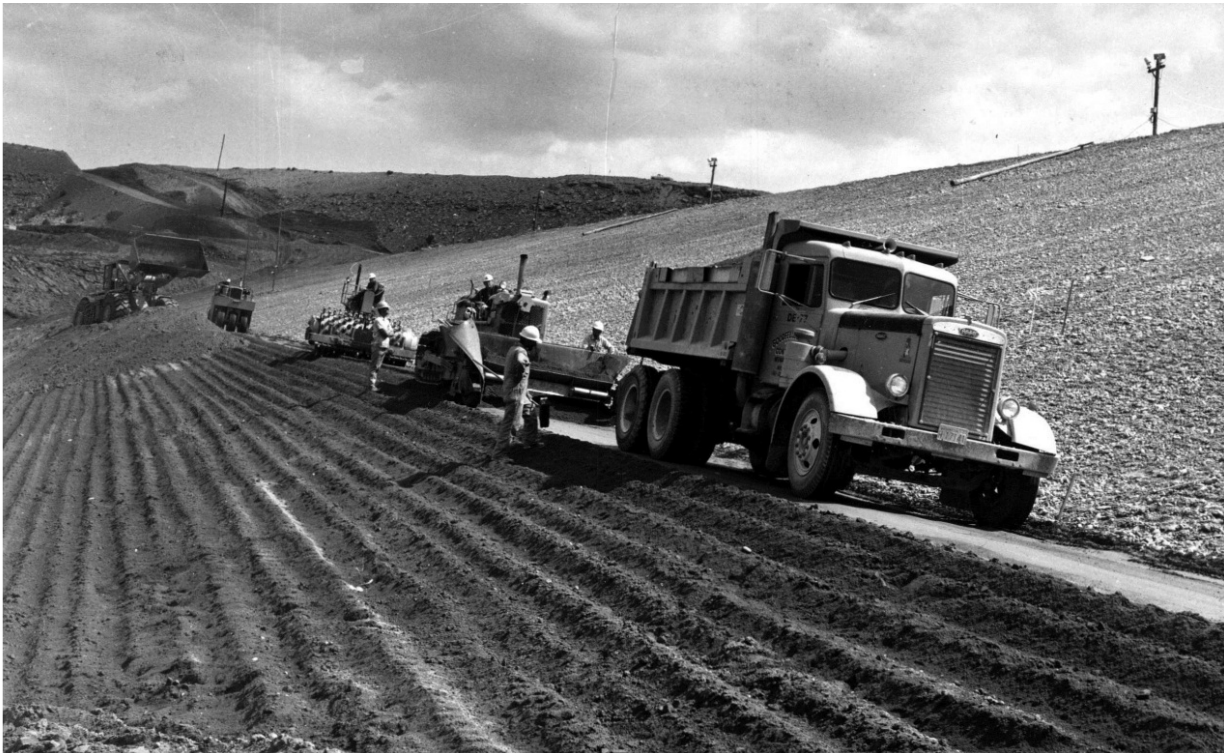
Figure 2.2.5.3.4-2. Placement of soil-cement slope protection, Starvation Dam, Utah.
