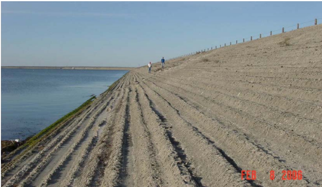
Figure 2.2.5.3.4-1. Soil-cement slope protection at Choke Canyon Dam, Texas.
