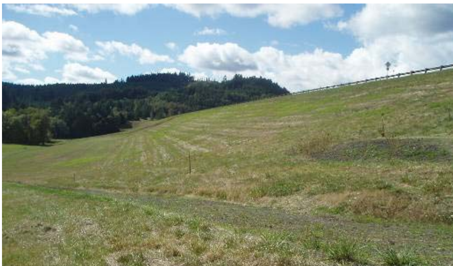
Figure 2.2.5.4-2. Vegetated slope protection on downstream slope of Scoggins Dam, Oregon.
