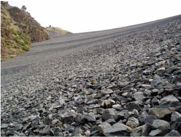
Figure 2.3.5.1-1. Rockfill on the downstream slope of New Melones Dam, California.
