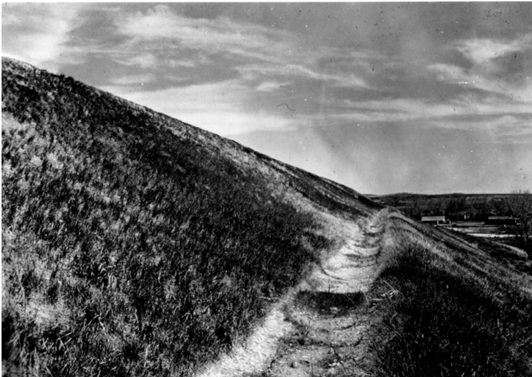
Figure 2.2.5.5-1. Contour ditch at Belle Fourche Dam, South Dakota.
