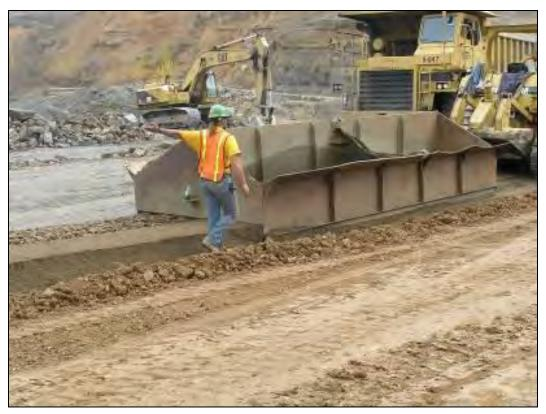
Figure 7-17. Towing spreader box.
