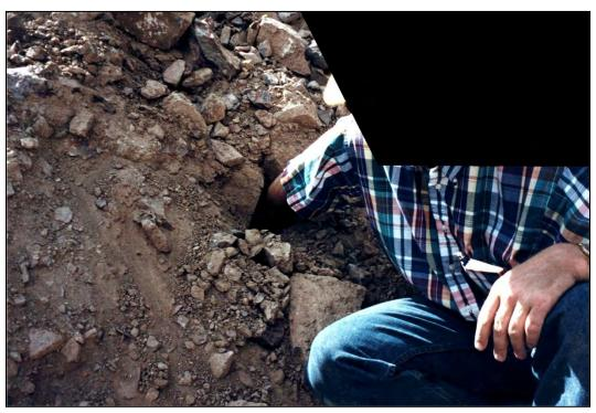
Figure 6-6. Open work present in the right abutment foundation of Ochoco Dam. The abutment consists of landslide debris.
