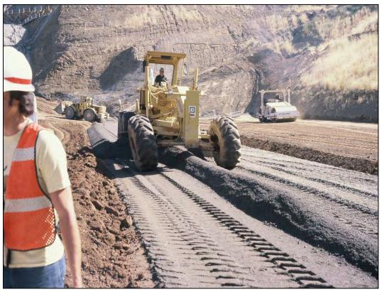
Figure 7-13. Spreading sand filter material.
