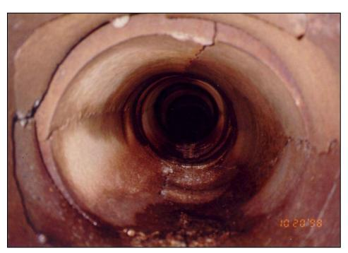
Figure 2-17. Interior view of a reinforced concrete pipe from the 1950s. Note that the pipe is overstressed, and cracks have formed at the crown and spring line. The pipe has also deformed to an oval shape. In the foreground, a joint can be seen and sand that passed through the joint.
