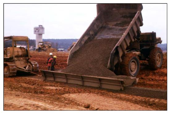
Figure 7-16. Dumping into spreader box.
