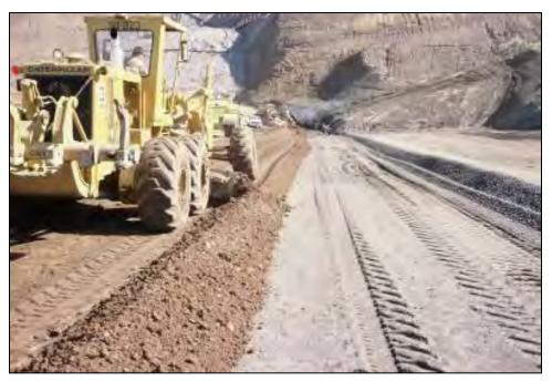
Figure 7-3. Windrowing impervious material adjacent to a filter/drain.
