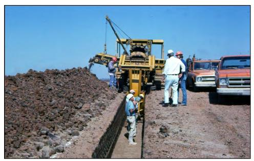
Figure 7-5. Trenching method – excavating trench.
