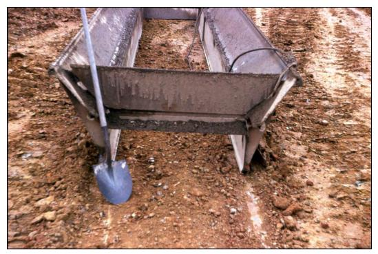
Figure 7-14. Basic single-bin spreader box.
