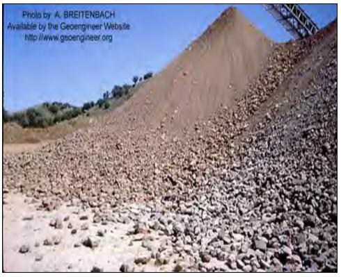
Figure 7-9. Segregation at high cone pile.
