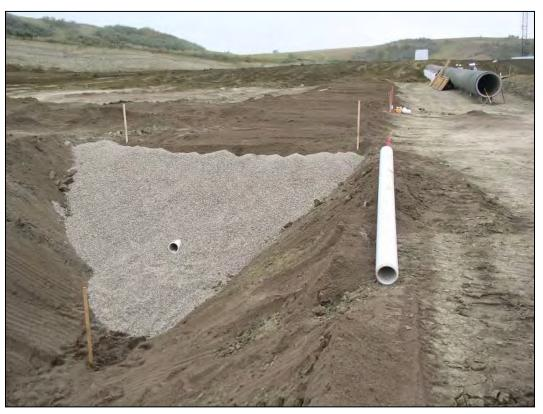
Figure 2-14. Trapezoidal foundation trench drain at toe of embankment. Coarse inner filter surrounds perforated PVC collector pipe and fine filter provides filter compatibility with foundation soils.
