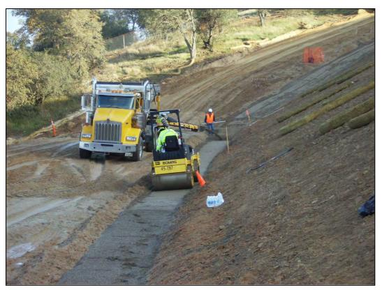
Figure 7-20. Truck conveyor delivering filter sand for the addition of a 4-ft-wide chimney filter to an existing embankment. Note that the material is uniformly placed from the conveyor, and no leveling is required. Dynamic compaction is provided by the roller shown in the foreground.
