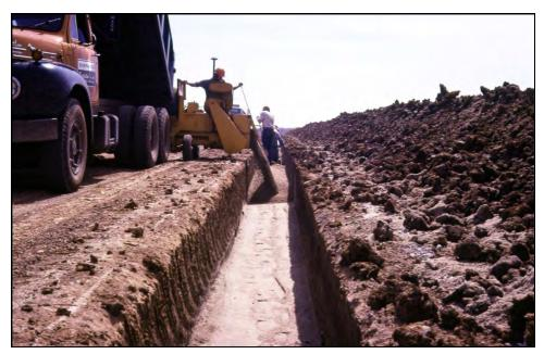
Figure 7-6. Trenching method – backfilling trench.
