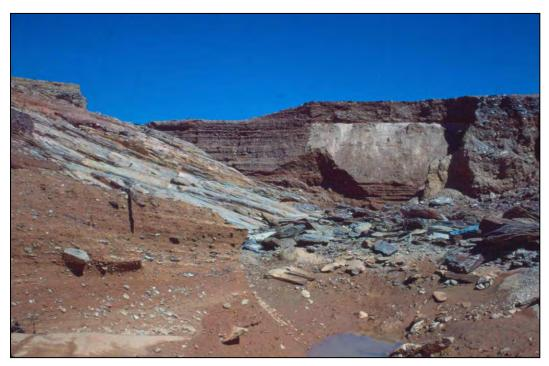
Figure E-3. Breach in left abutment viewed in upstream direction. Right abutment is to left foreground. Overtopping flow washed the embankment and overburden down to clean rock.
