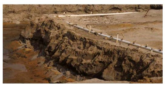
Figure L-32-1.--Well points used to dewater excavation below the water table.
