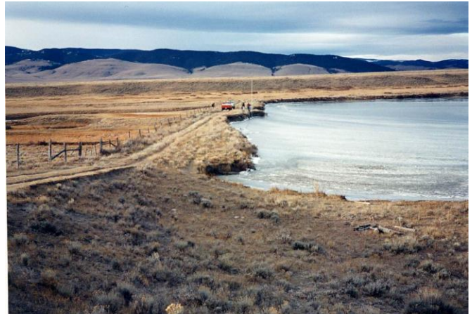
Figure 1: Erosion of a small embankment dam in Montana caused by wave action.
