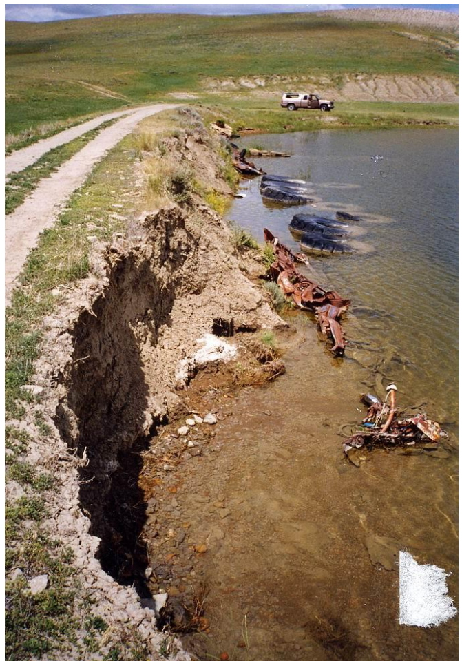
Figure 2: Erosion of a small embankment dam in Montana caused by wave action.
