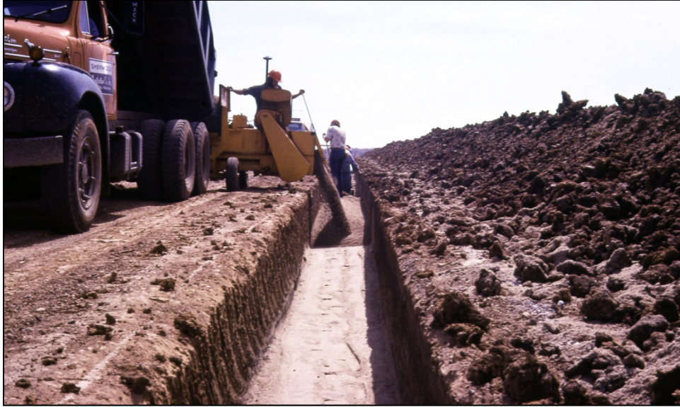
Figure 5.8.2.3-3. Trenching method – backfilling trench.
