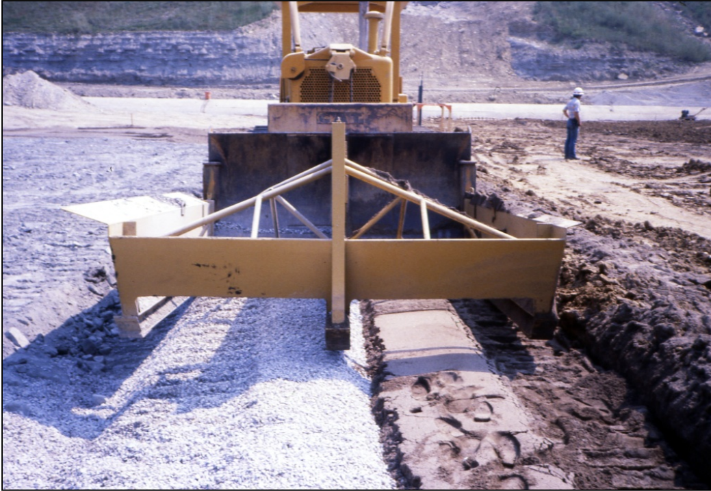
Figure 5.8.2.5.2-6. Double-bin spreader box fitted to dozer (end view).
