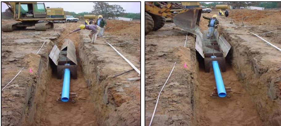
Photo 5.2.3.2.1-1. Rectangular cross section foundation trench drain with gravel filter (envelope) surrounding perforated collector pipe and fine sand filter in primary part of drain. Boxes are contractor’s innovative idea of placing the coarse filter around the pipe. By closing the top of the box, fine drain fill can be placed and kept separated from the coarse drain zone.
