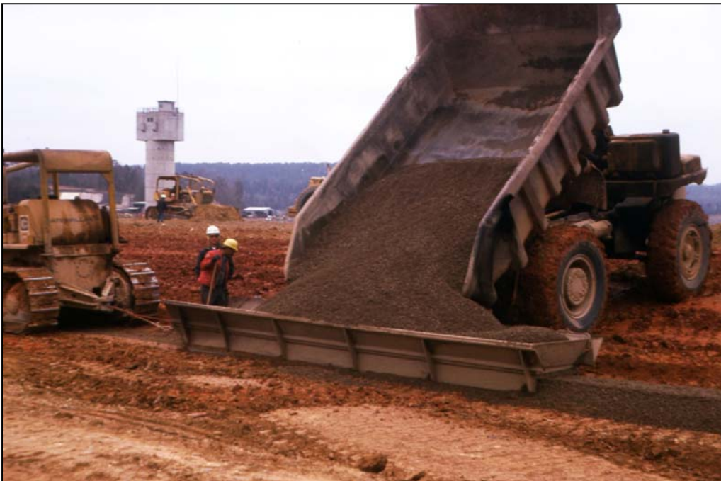
Figure 5.8.2.5.2-3. Dumping into spreader box.
