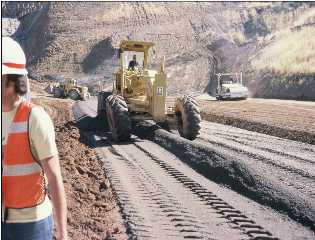
Figure 5.8.2.5.1-1. Spreading sand filter material.
