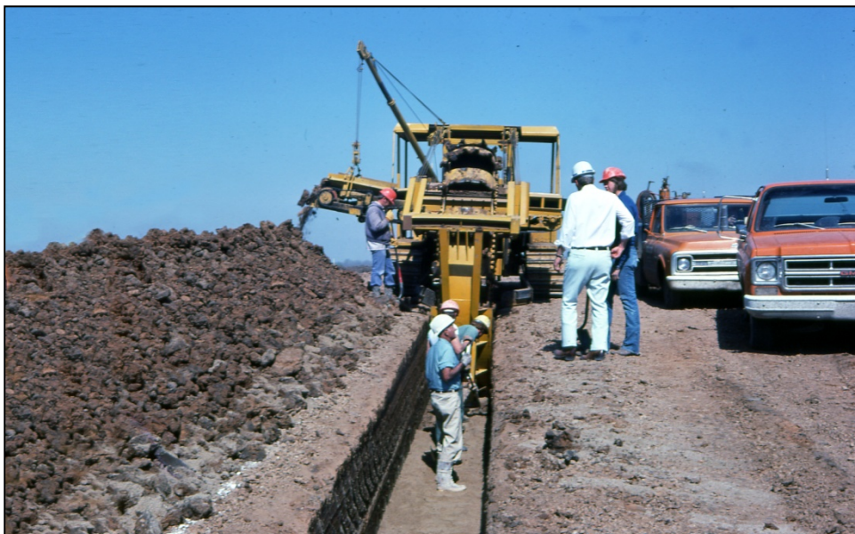
Figure 5.8.2.3-2. Trenching method – excavating trench.
