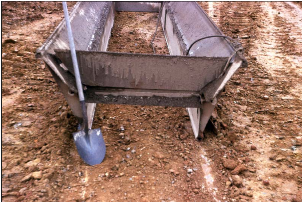
Figure 5.8.2.5.2-1. Basic single-bin spreader box.
