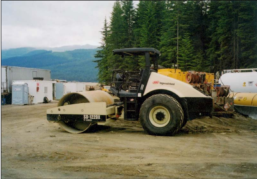
Figure 5.8.5.1.1-2. Single-drum vibratory roller.
