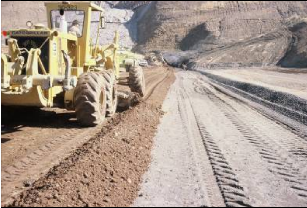
Figure 5.8.2.2-2. Windrowing impervious material adjacent to a filter/drain.
