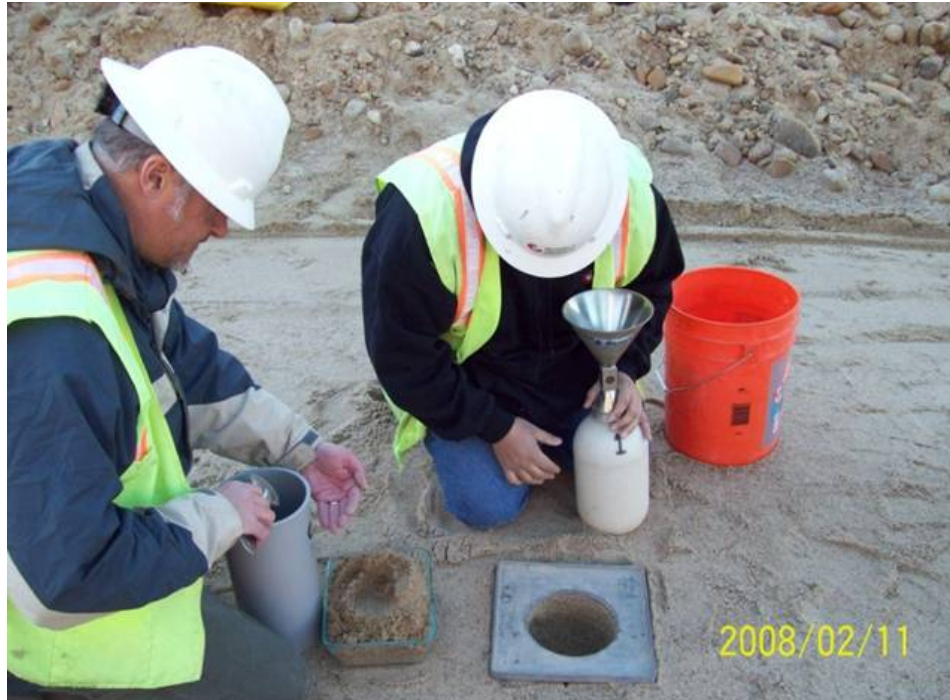
Figure 5.8.7.2.1-1. 'Sand Cone Test' being performed in a sand blanket filter.
