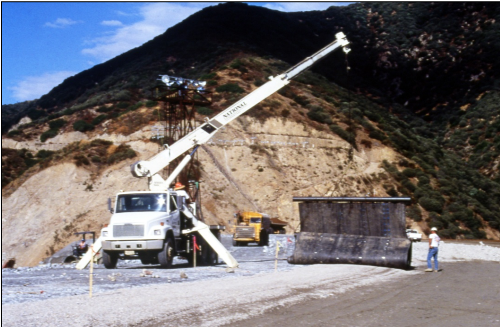
Figure 5.8.6.1.2-3. Placement of geomembrane at crossing over a chimney filter and drain.
