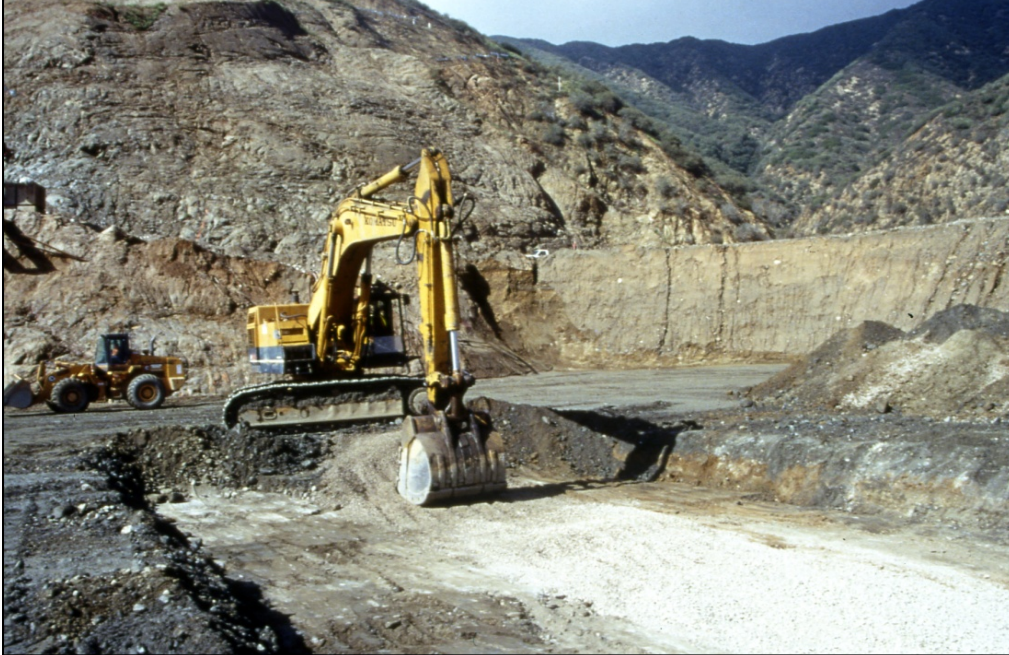
Figure 5.8.6.1.2-2. Excavation of filter material under equipment crossing.
