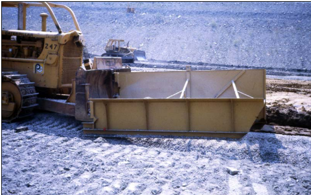
Figure 5.8.2.5.2-5. Double-bin spreader box fitted to dozer (side view).
