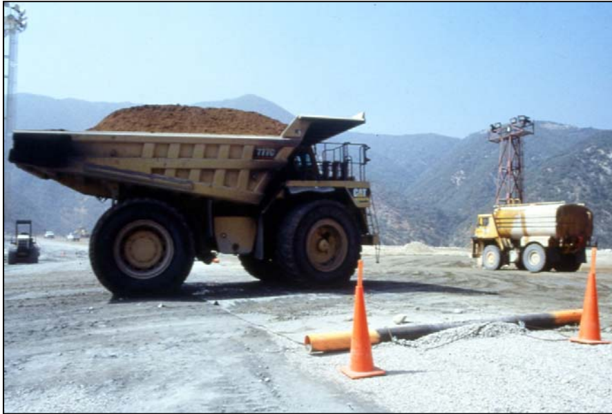
Figure 5.8.2.4-1. Large end-dump truck using an equipment crossing over a chimney filter.
