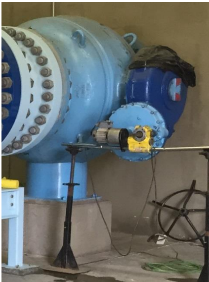
Photo 6: Ball Valve with Actuator
