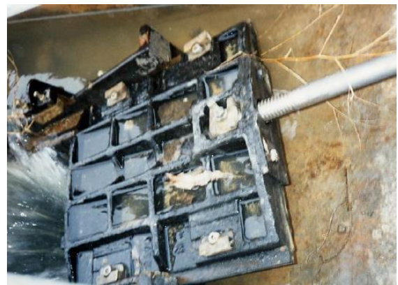
Photo 4: Angled Intake Sluice Gate Parallel with Upstream Face of Dam
