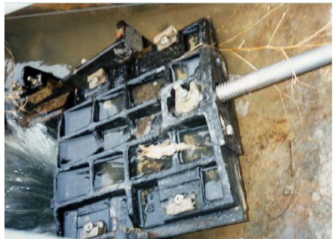
Photo 3: Angled intake gate parallel with upstream face of dam
