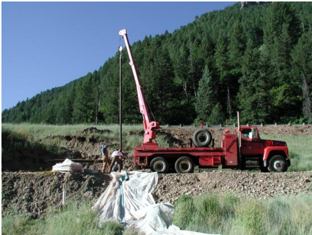
(a) Crane truck support vehicle
