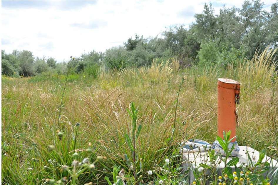
Figure 21.9.4-3. Typical above ground portion of a piezometer (photo by W. Robert Talbot).
