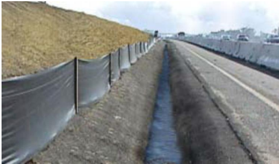
Figure 21.8.6.1-1. Lined trench/ditch at the base of a slope. Slope erosion is also controlled by a mulch covering on the slope and a silt fence near the toe of the slope (photo from State of California Department of Transportation, 2003).
