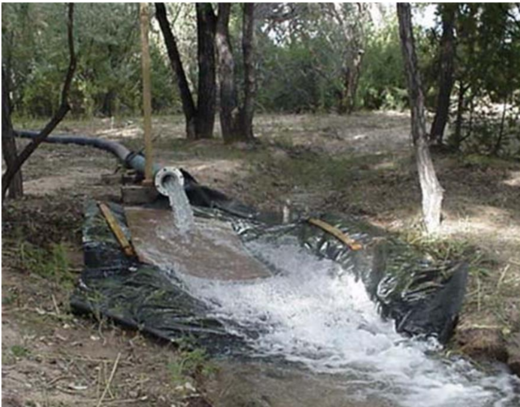
Figure 21.9.3-1. Erosion protection at discharge point. Discharge is reported as 1,000 gpm (Collector Wells International, Inc., 2002, San Ildefonso Pueblo Demonstration Collector Well, Rio Grande, New Mexico).
