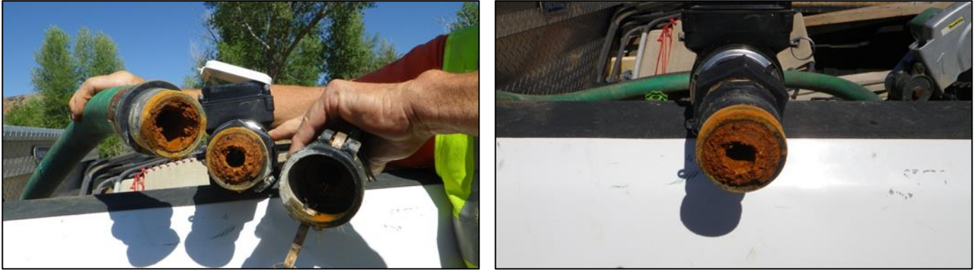
(a) Discharge lines installed about 1 year apart
