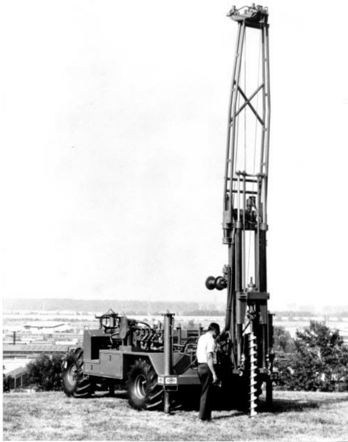
Figure 21.9.2-1. Continuous-flight auger mounted on an all-terrain carrier (figure 2-22 in Reclamation, 1990a).
