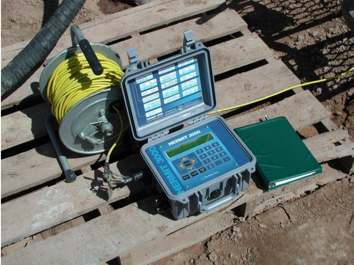
Figure 21.8.10-7. In-Situ Hermit 3000® data logger and “Rite-in-the-Rain” field notebook. Data logger is connected to a dedicated pressure transducer in a pumping well via the yellow, vented cable. Drawdowns are recorded manually every hour, and the corresponding data logger readings are manually recorded in case of data logger or transducer failure (National Desalination Research Facility, Alamogordo, New Mexico, photo by W. Robert Talbot).
