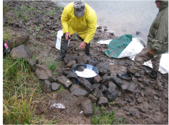
Photo 6: Final application of grout, contained within pipe (Fish Lake)
