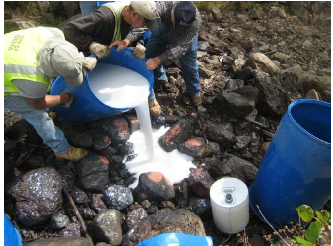
Photo 4: Application of chemical urethane grout (Big Battlement Dam)
