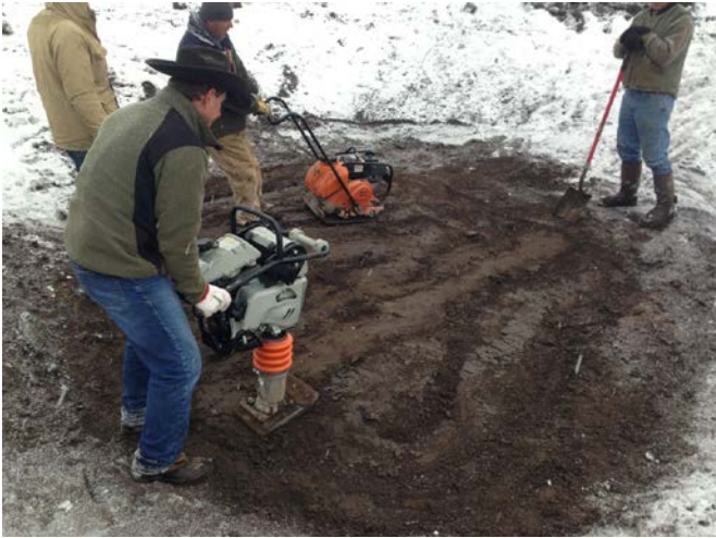
Photo 8: Compaction of clay layer at Lake Ann, CO
