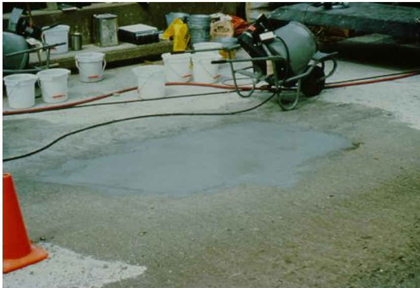
Figure 96. Protecting the polymer concrete until it gets hard.
