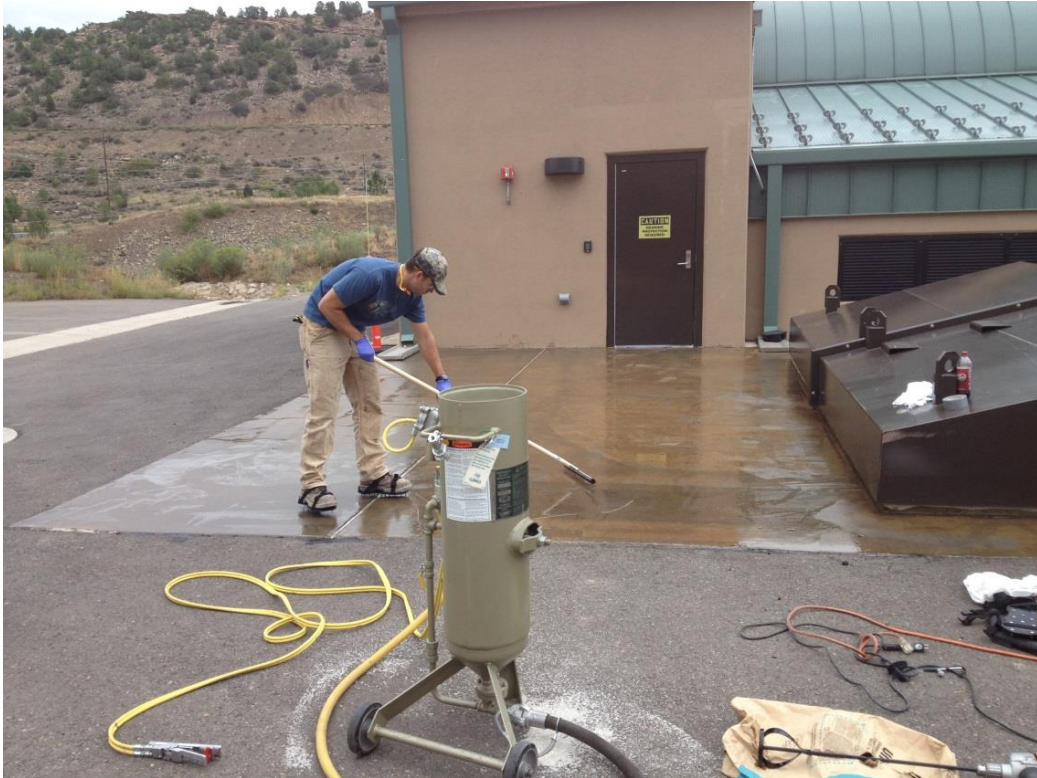
Figure 80. Application of an epoxy sealer to a pumping plant deck.
