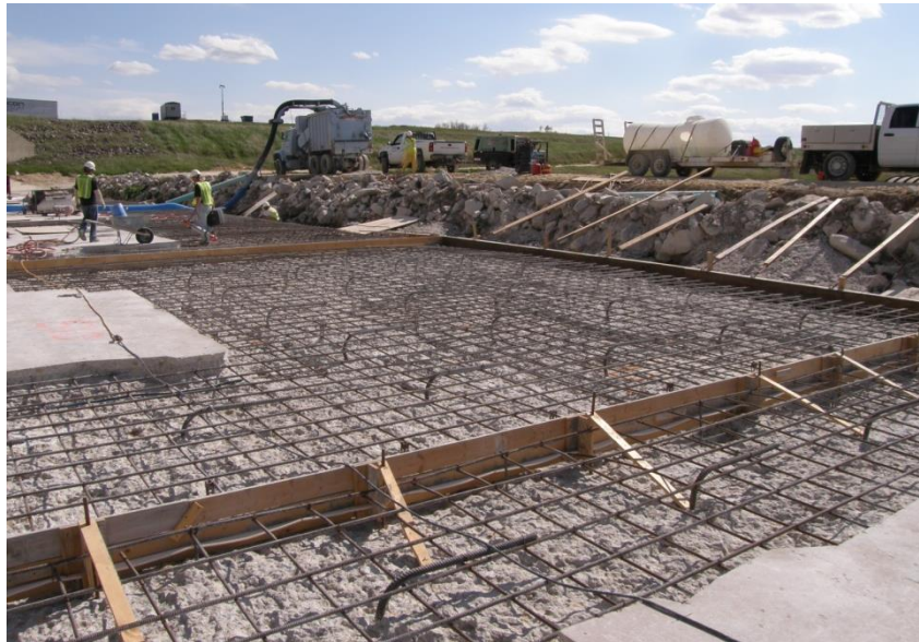
Figure 31. A properly prepared area for repair to a spillway approach apron.
