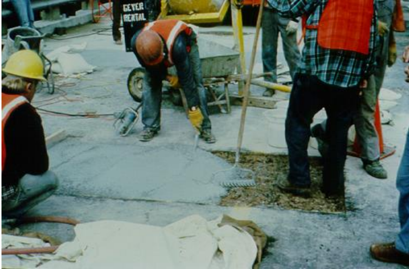
Figure 95. Consolidating polymer concrete with a vibrator.
