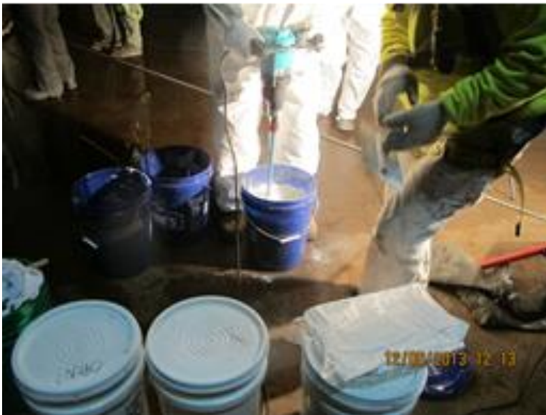
Figure 92. Mixing epoxy mortar ingredients in buckets.
