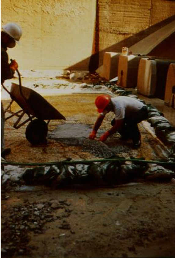
Figure 93. Placing polymer concrete to repair shallow damage to a stilling basin.
