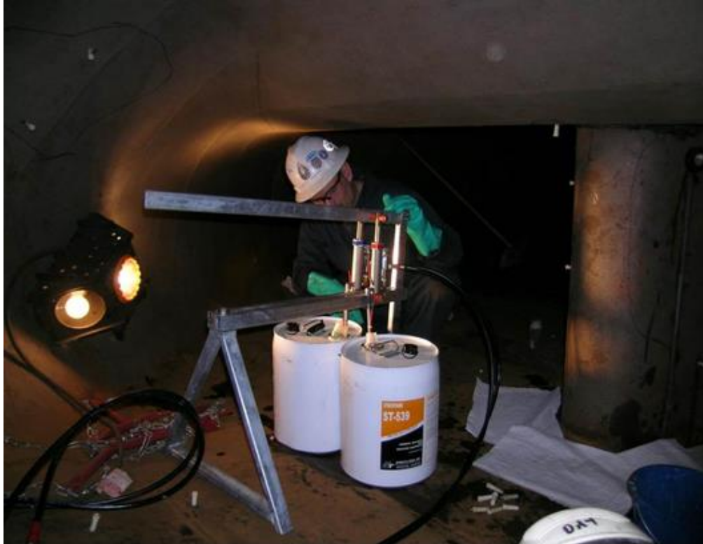
Figure 121. Hand-operated pump used to inject resin in difficult access areas.
