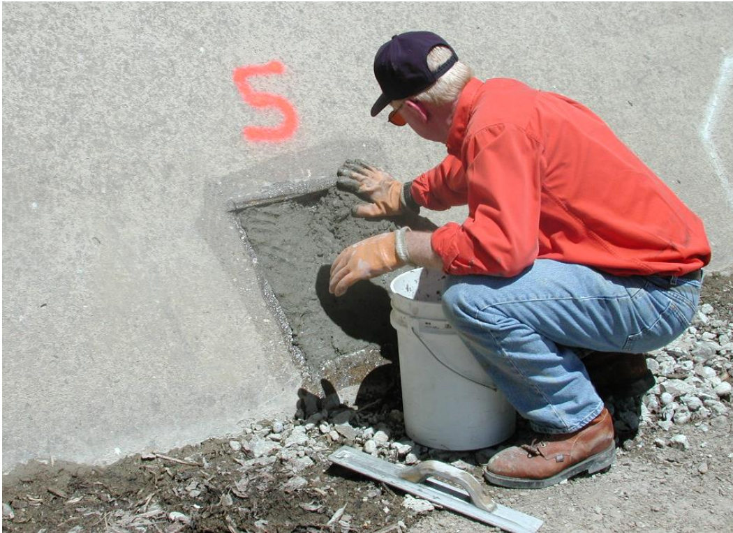
Figure 100. Applying a stiff repair mortar using hand packing.
