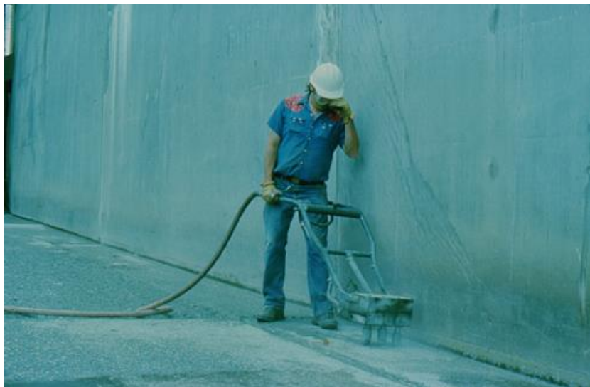
Figure 27. A scabbler used to remove concrete.
