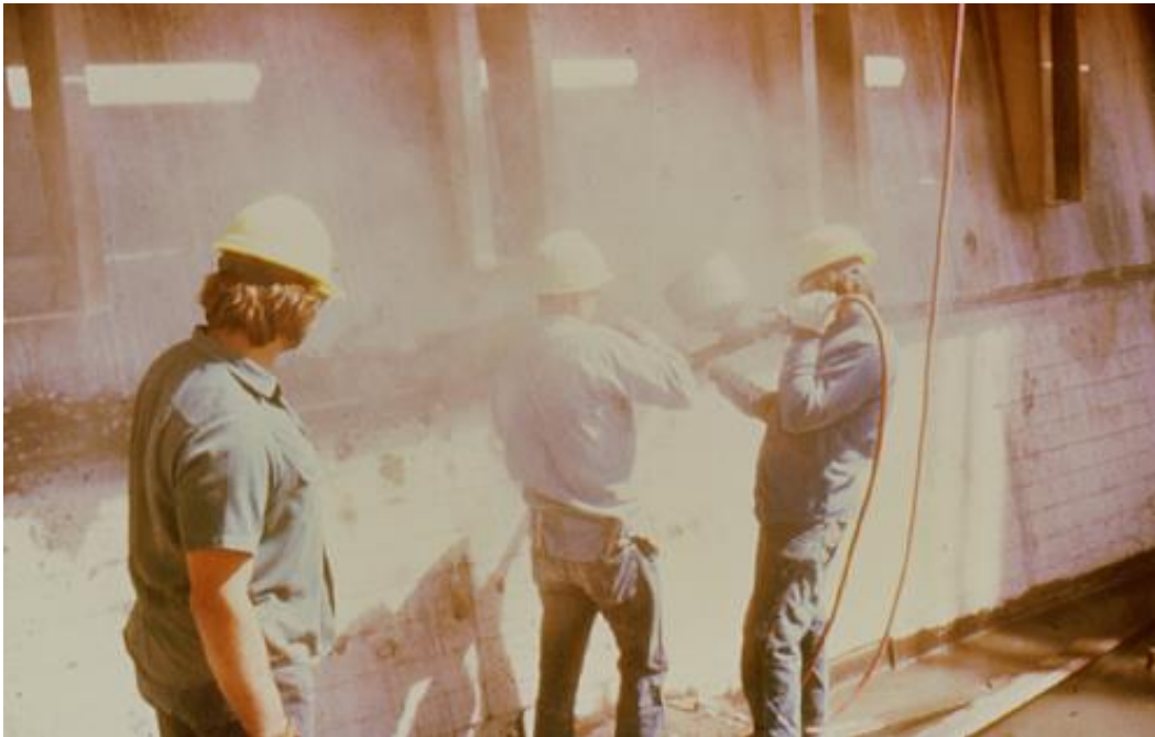
Figure 87. Using low-pressure spray equipment to apply Portland cement mortar.
