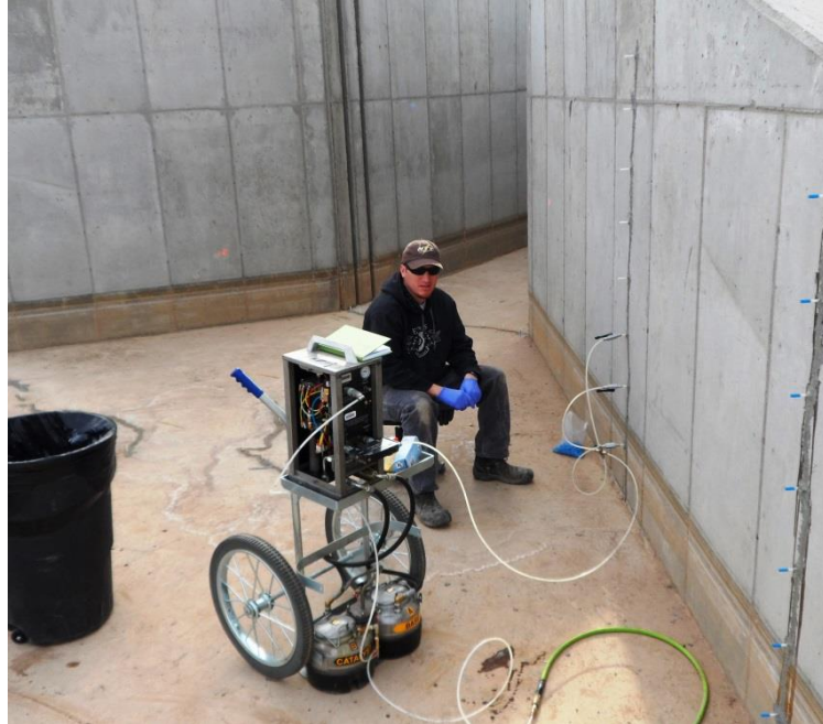
Figure 124. Simultaneous injection of multiple injection ports for epoxy injection.
