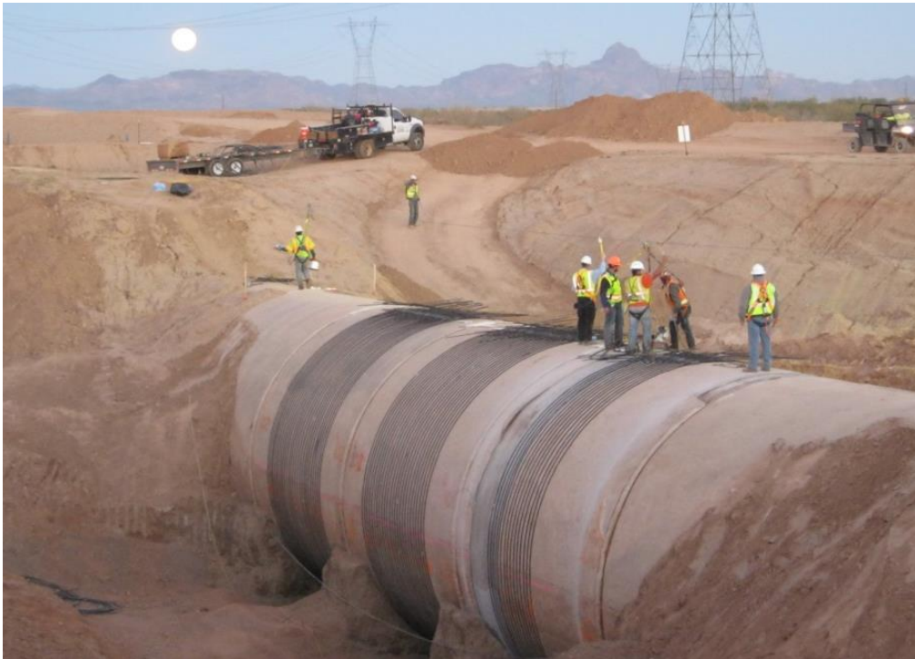
Figure 107. Adding additional reinforcement to the exterior of a large-diameter siphon.
