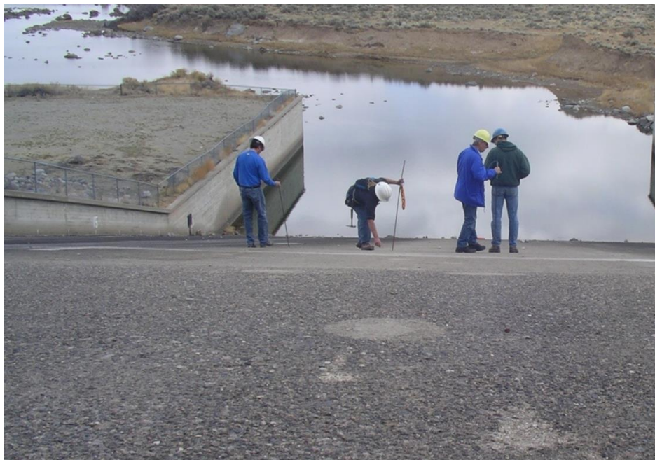
Figure 7. Inspecting a spillway floor using steel bars to sound the concrete. The soundings indicated delaminations in the spillway floor.
