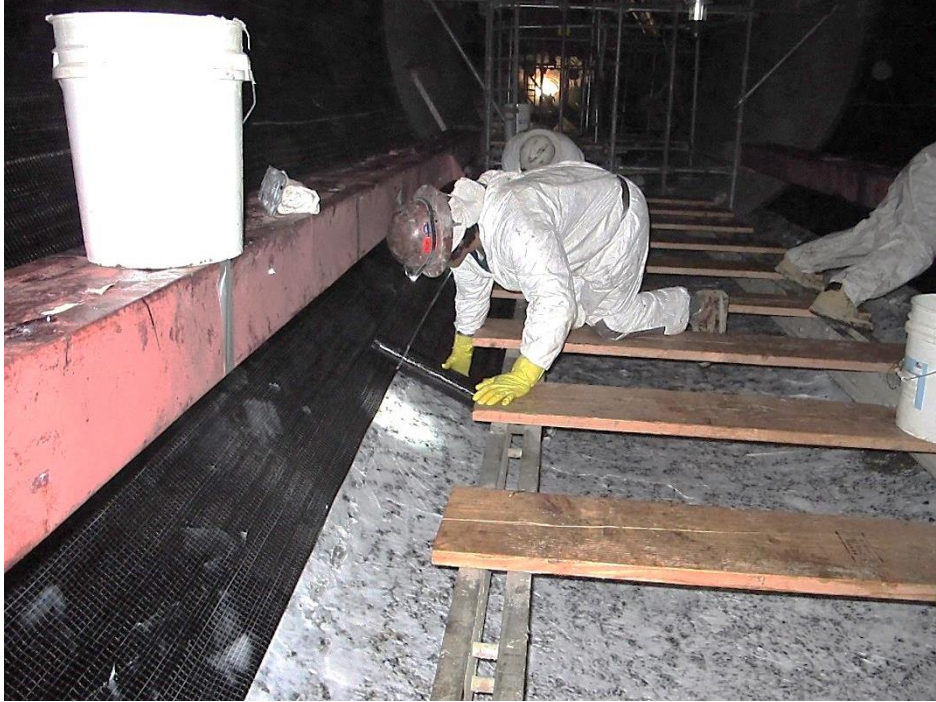
Figure 108. Installing carbon fiber reinforced polymer to repair a large concrete pipe.
