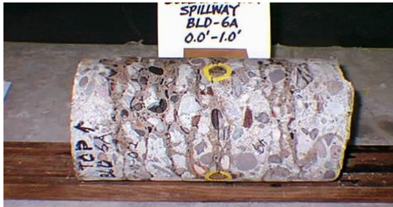
Figure 49. Freeze-thaw deterioration in a spillway slab occurring below the exposed surface, due to moisture and temperature gradients.
