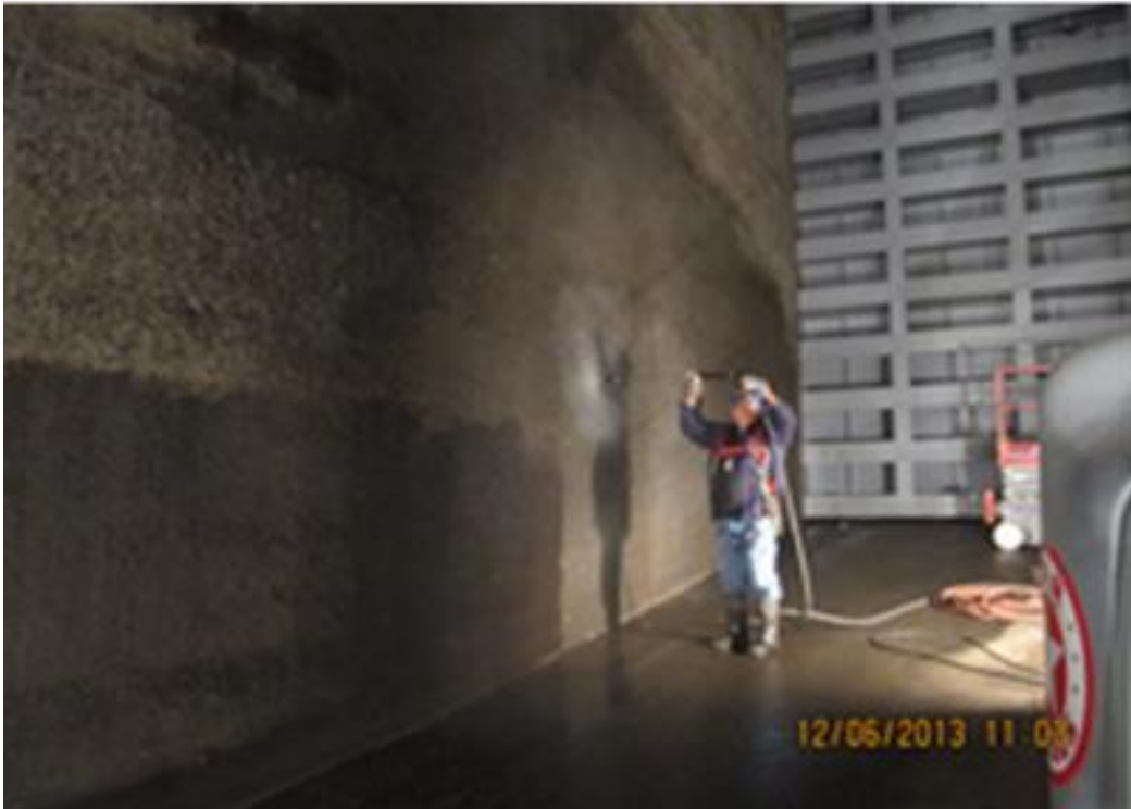
Figure 32. Using water jetting for secondary cleaning (4,000 psi).
