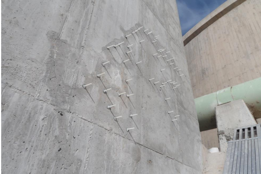
Figure 113. Ports glued to the face of cracks prior to epoxy injection.
