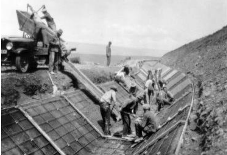
Figure 5. Early concrete canal lining. Horse and buggy transporting gave way to central batch plants and the first motorized transporting buggies. Still, the concrete placing and compacting processes were performed by laborers with shovels (Bureau of Reclamation historical photographs).
