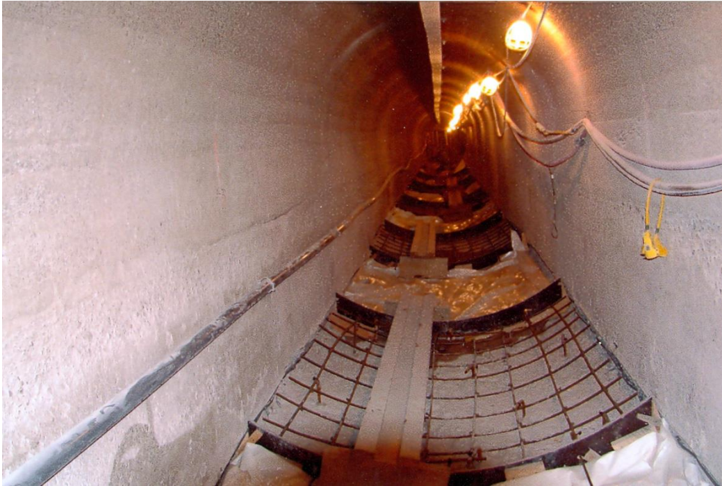
Figure 101. An outlet works repair being prepared for replacement concrete.
