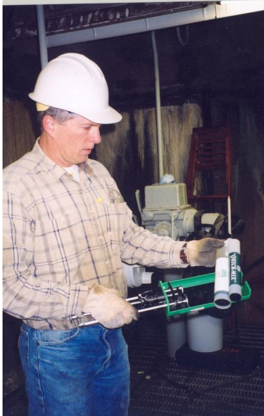
Figure 118. Two-component cartridge system for injecting resin into cracks.
