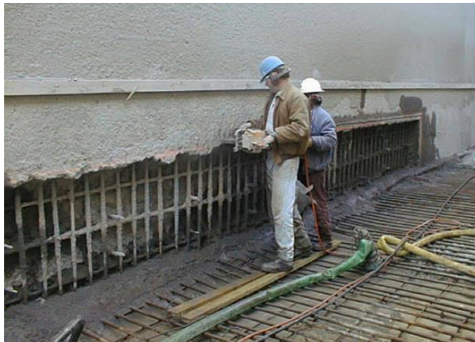
Figure 19. Saw cutting the perimeter after hydrodemolition removed most of the concrete.
