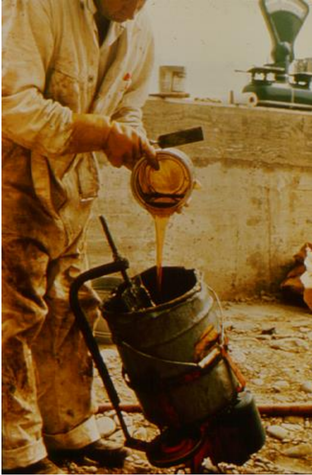
Figure 91. Using a simple bucket mixer to mix epoxy resin.
