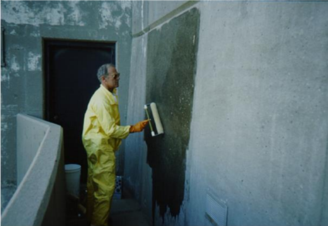
Figure 82. Application of a siloxane sealing compound.
