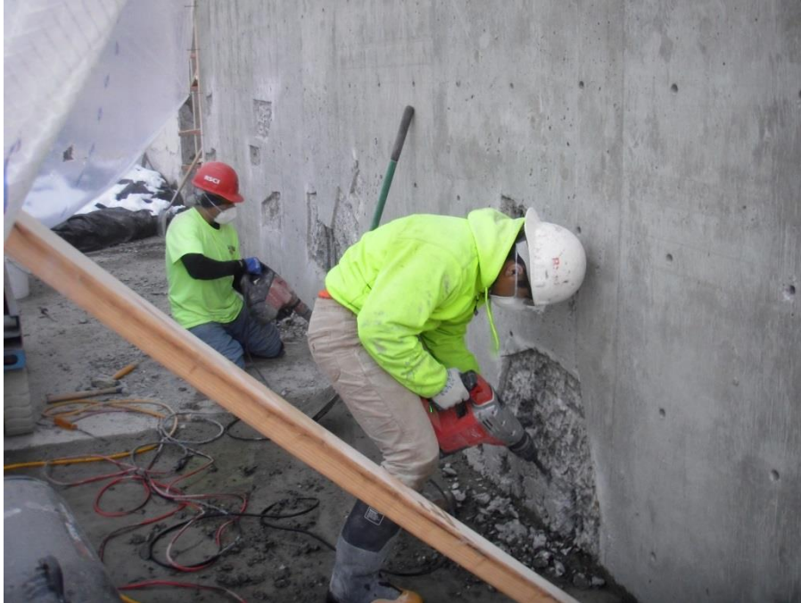
Figure 24. Using a small electric chipping hammer to remove damaged concrete.
