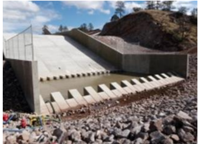
Figure 11: Lined Spillway Chute (Concrete)
