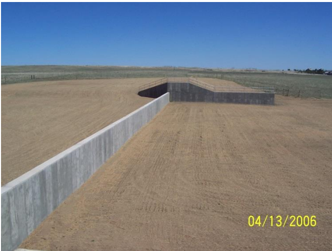
Figure 5: Sharp Crested Weir
