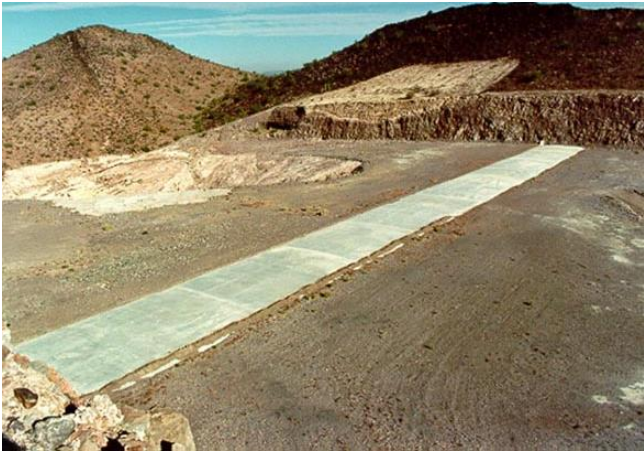
Figure 4: Concrete Control Sill
