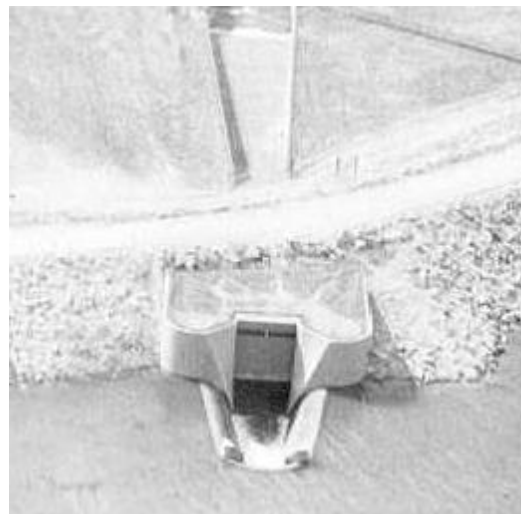
Figure 10: Bathtub Crest Structure (Reclamation 1987)
