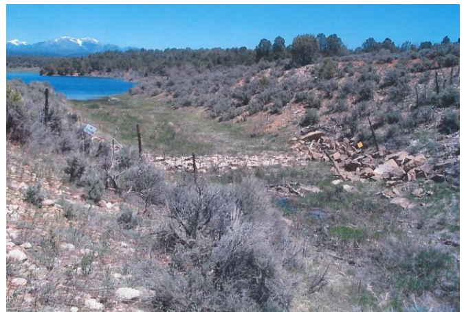
Figure 13: Unlined Spillway Chute
