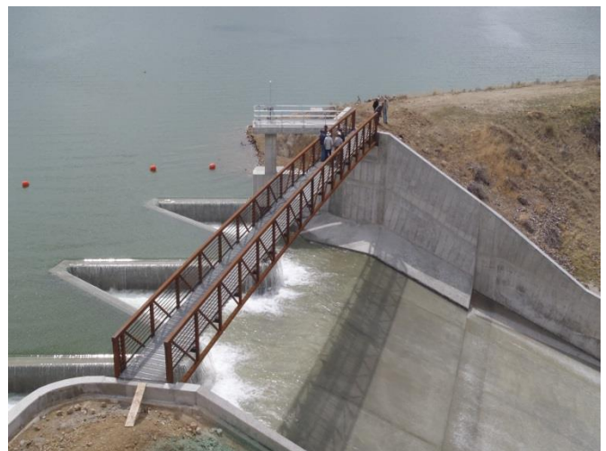
Figure 6: Labyrinth Weir
