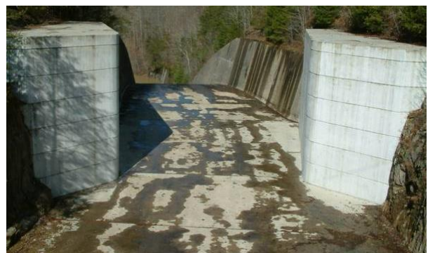
Figure 3: Broad Crested Weir
