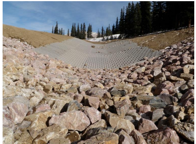
Figure 12: Lined Spillway Chute (Articulated Concrete Blocks and Riprap)
