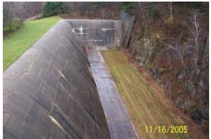
Figure 9: Side Channel Spillway
