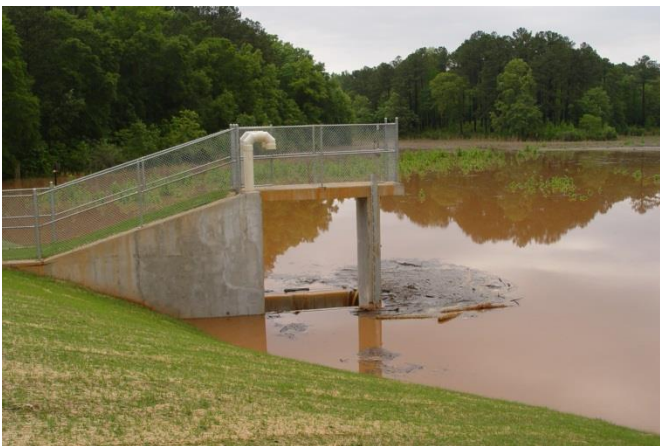
Figure 8: Drop Inlet
