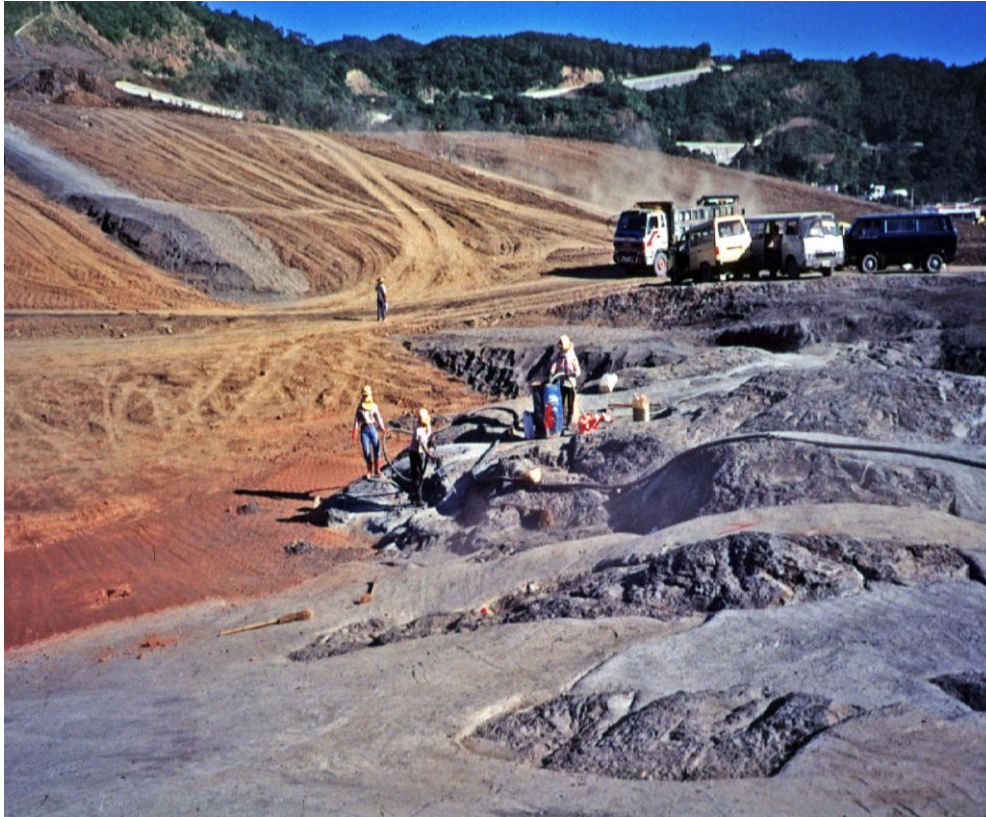
Figure 3.2.6.3-4 Feathering at the ends of concrete placements should not be permitted. The edges of concrete should be sloped no flatter than 45 degrees.
