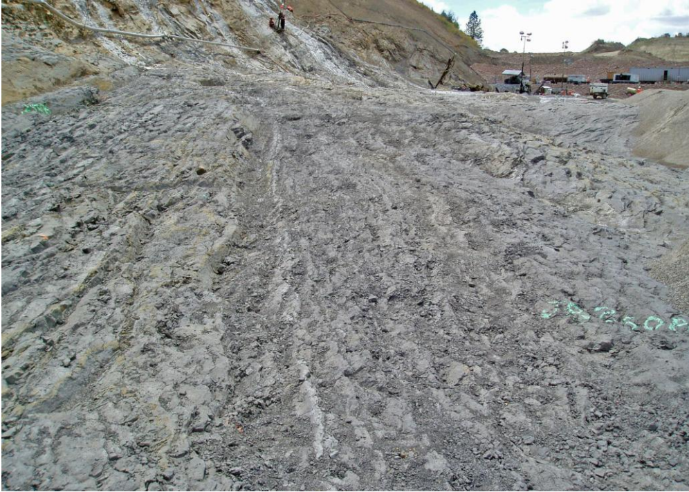
Figure 3.2.4.2-6 Ridges Basin Dam. Foundation after stripping and before cleanup.
