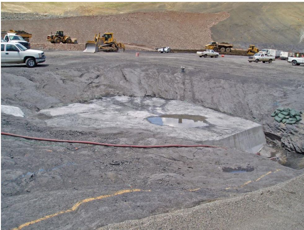
Figure 3.2.6.6-4 Ridges Basin Dam. Foundation dental concrete. Sometimes a dental concrete slab is a mass placement.
