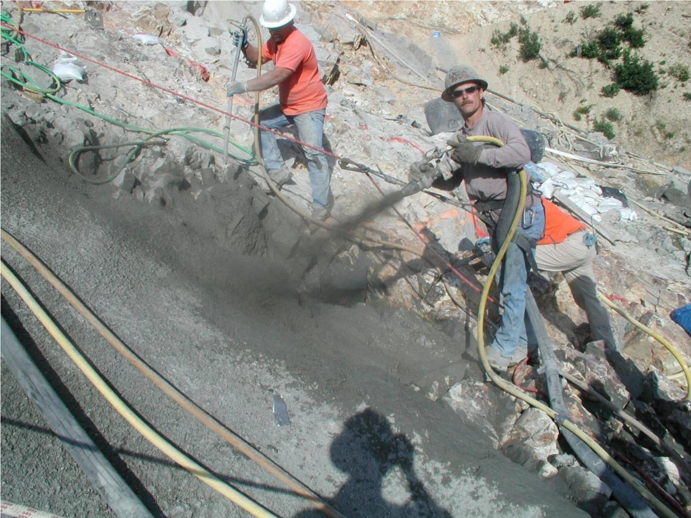
Figure 3.2.6.5-1 Shotcrete application.
