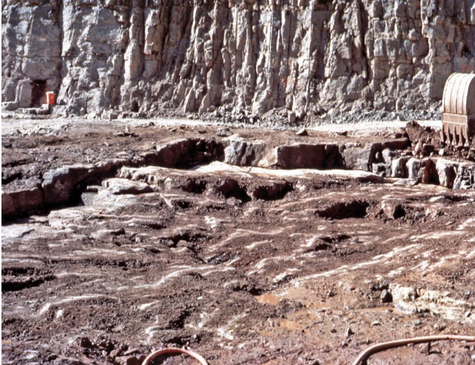
Figure 3.2.6.6-6 Upper Stillwater Dam. After stripping and before cleanup.
