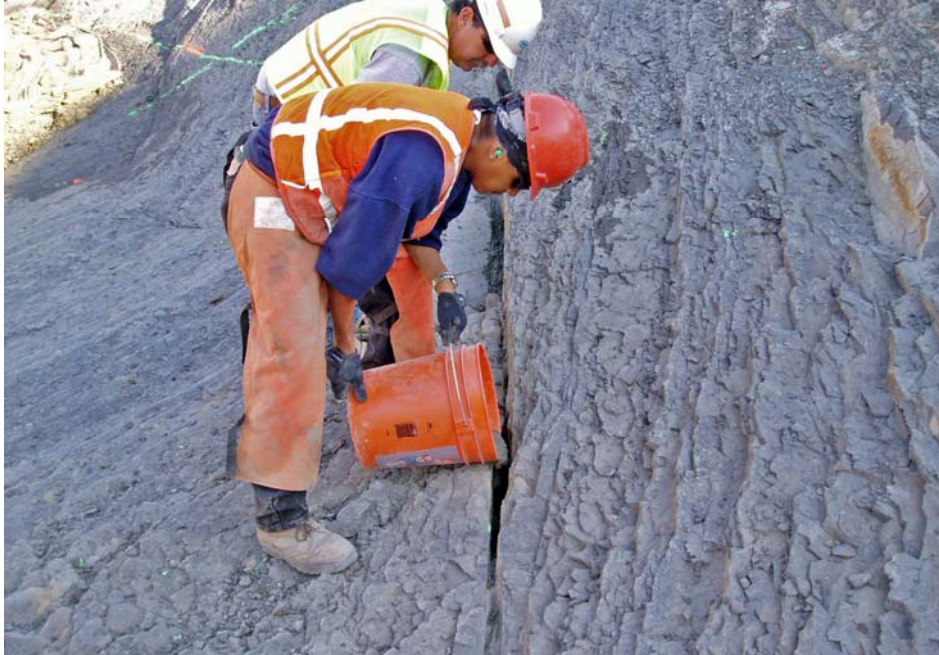
Figure 3.2.6.4-1 Ridges Basin Dam. Slush grout application in an open, cleaned joint.
