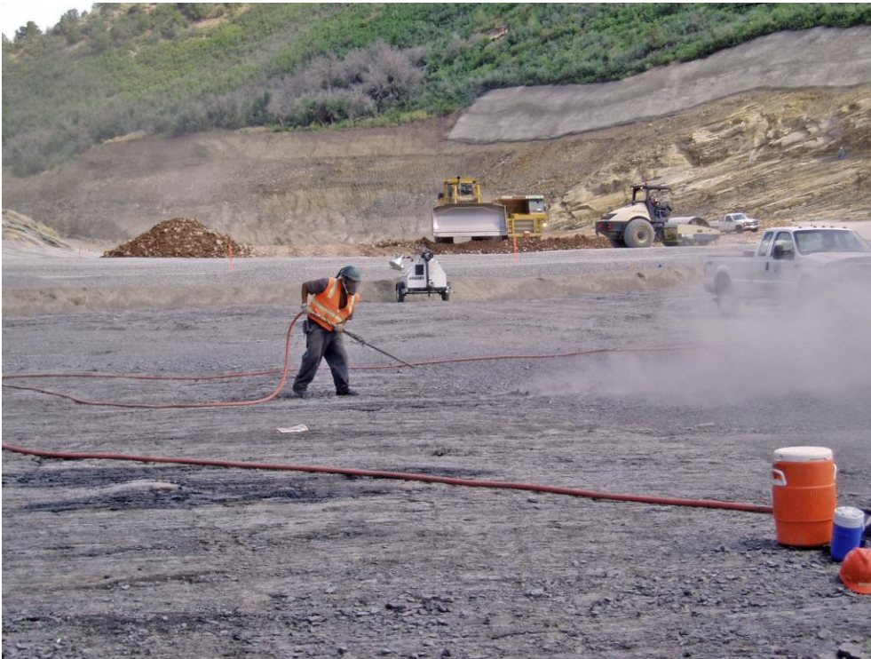
Figure 3.2.4.2-7 Ridges Basin Dam. Foundation cleanup using compressed air blow pipe.
