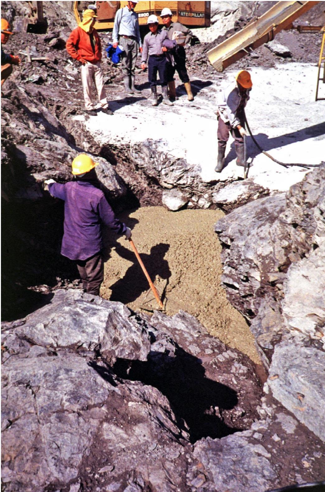
Figure 3.2.6.6-2 Treating foundation with dental concrete.
