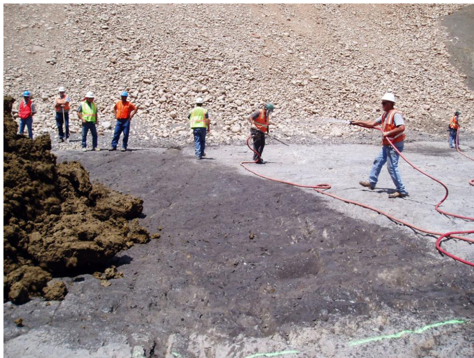
Figure 3.4.2-5 Ridges Basin Dam. Final foundation cleanup, wetting, and placing first lift.
