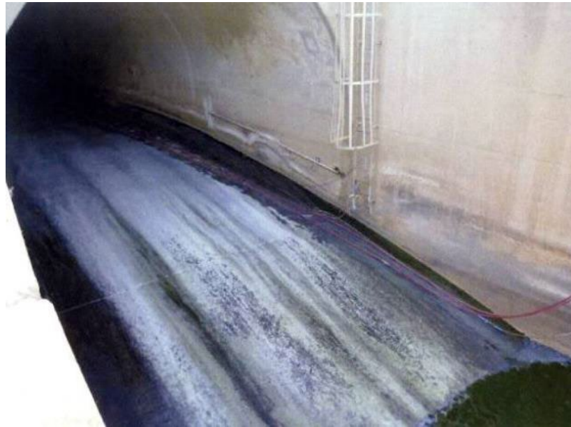
Outlet works chute.
