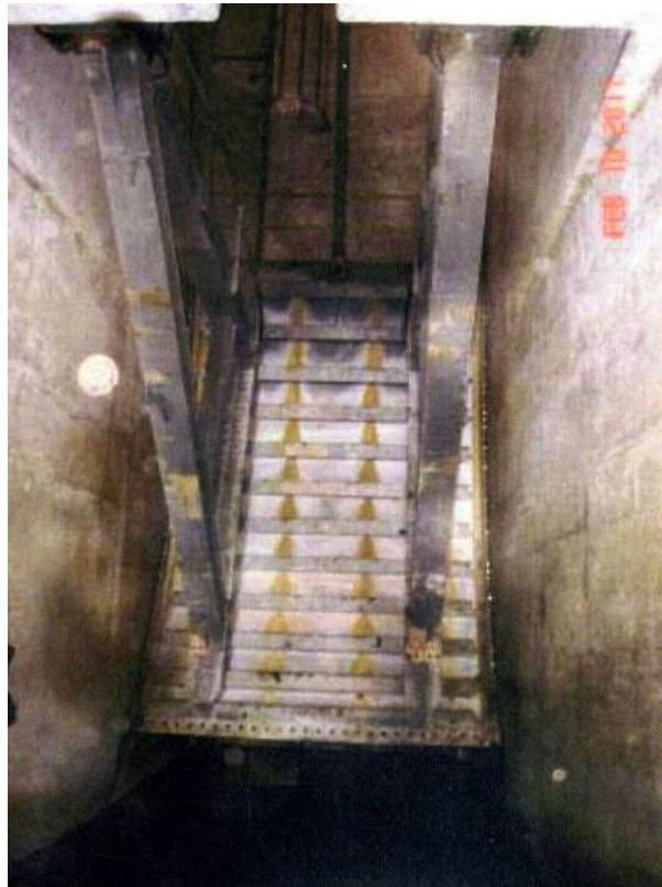
Figure 4.9.1.1-16. Top-seal radial gate.
