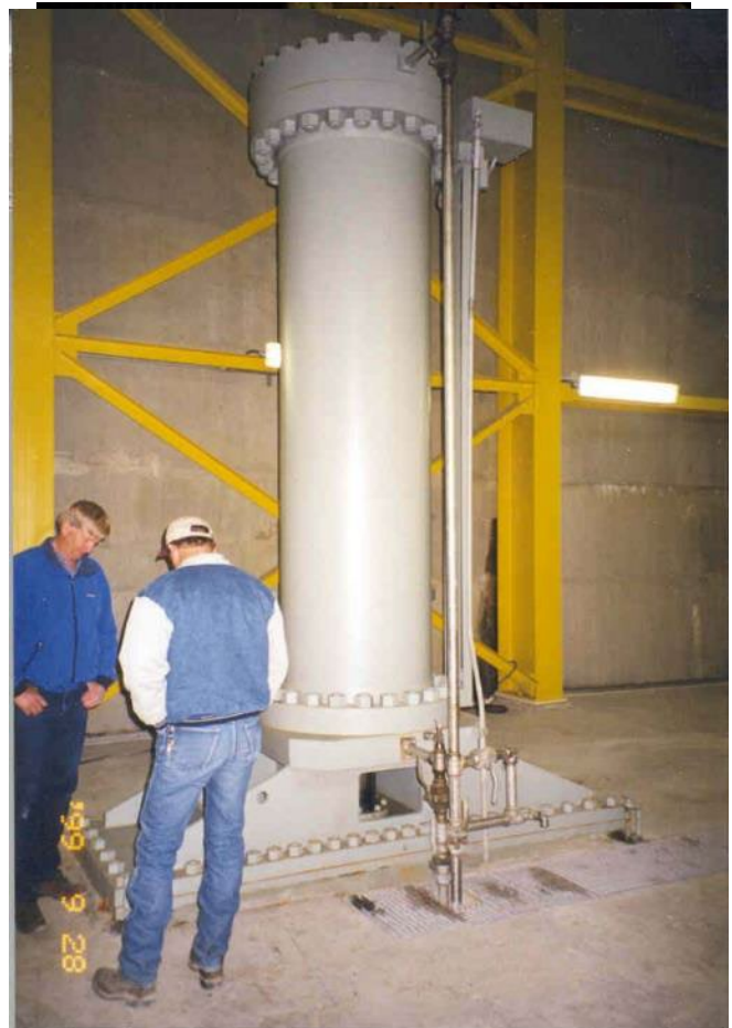
Figure 4.9.1.1-10. Outlet gate.
