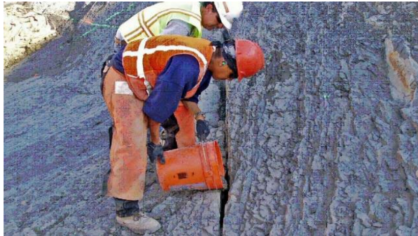
Figure 4.7.2.1.2-1. Slush grouting.
