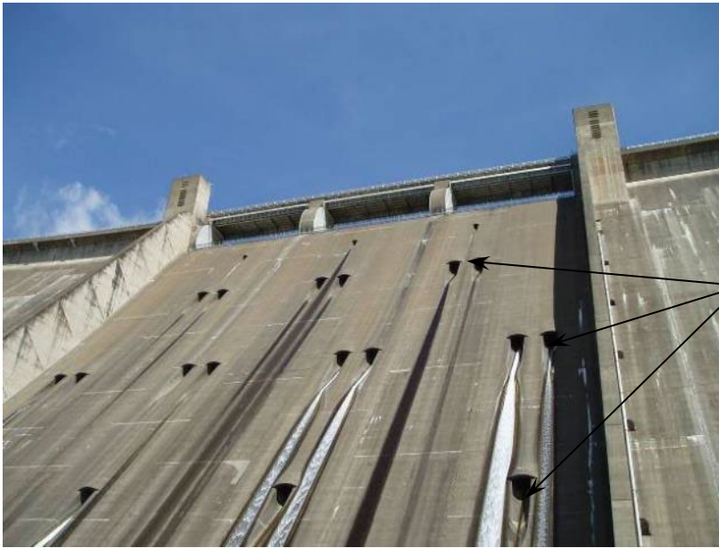
Combined outlet works and spillway chute.
