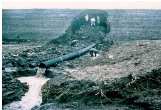
Internal erosion induced dam failure resulting from corrugated metal pipe that rusted through and exposed adjacent embankment to erosive flows (unknown dam).
