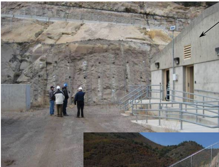
Profile view of rock slope excavation and rock bolts layout at the downstream outlet works portal.
