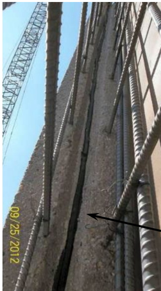
Figure 4.8.6.2-1. Retrofit and strip waterstops.
