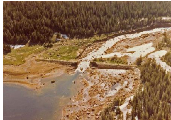
1982 internal erosion induced dam failure resulting from pressurized flow exiting the outlet works into the surrounding embankment material (Lawn Lake Dam, Colorado).
