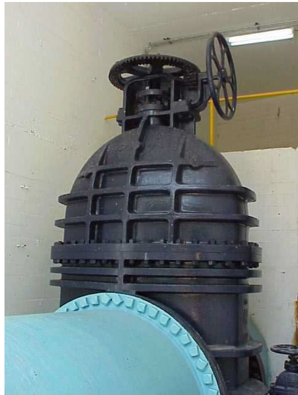
Figure 4.9.1.1-6. Gate valve.
