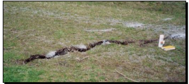
Photo 11: Transverse crest crack (ASDSO)
