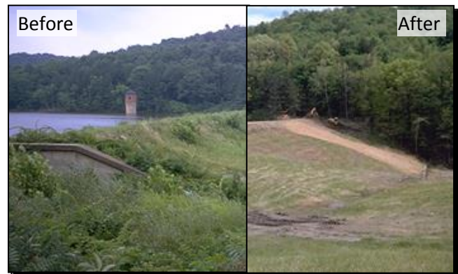
Photo 3: The importance of mowing before an inspection.
