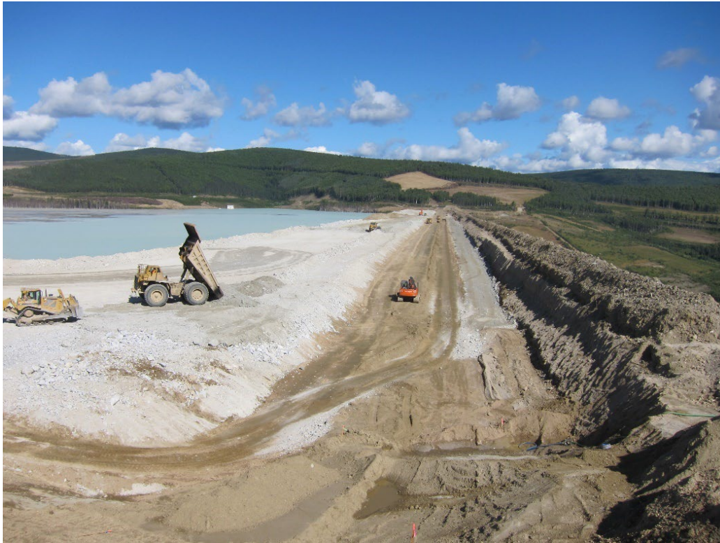
Figure III-5. Zoned-fill tailings dam constructed by downstream method at hard rock mine under transition to the modified centerline method for raises (photo by Chandler Engel)
