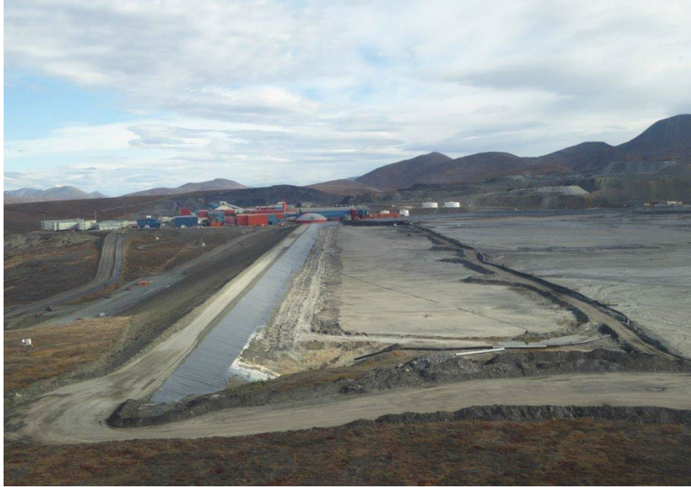
Figure III-4. Tailings dam at hard rock mine constructed by downstream method (photo by Al Ott)
