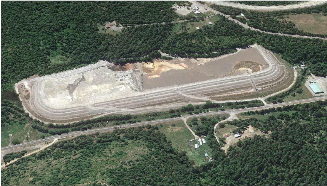
Figure III-2. Tailings dam at hard rock mine constructed by the upstream method (Google Earth, 2017)
