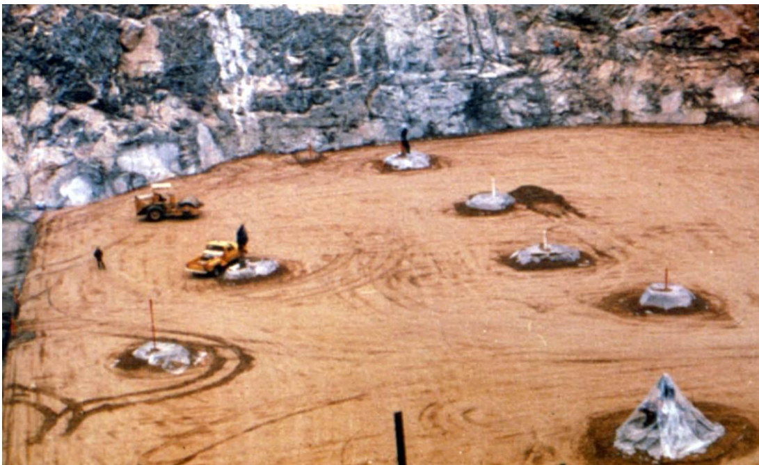
Figure 11.2.5.5-1. Protective mounds around instrumentation installations at an embankment dam under construction.
