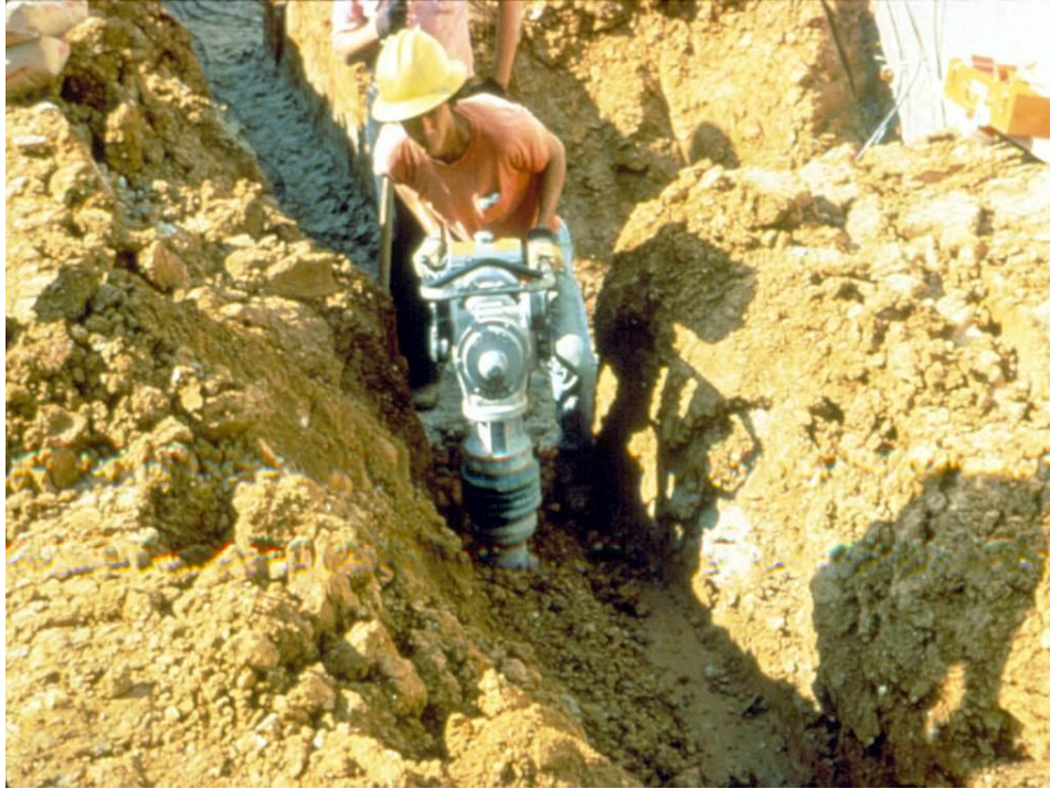
Figure 11.10.2-1. Special compaction efforts taking place in an instrumentation cable trench.
