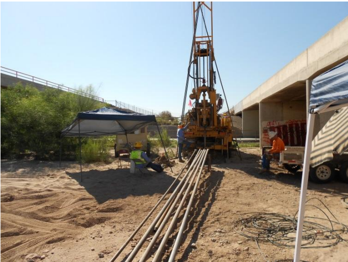
Photo 4. Mud Rotary Drill Rig
