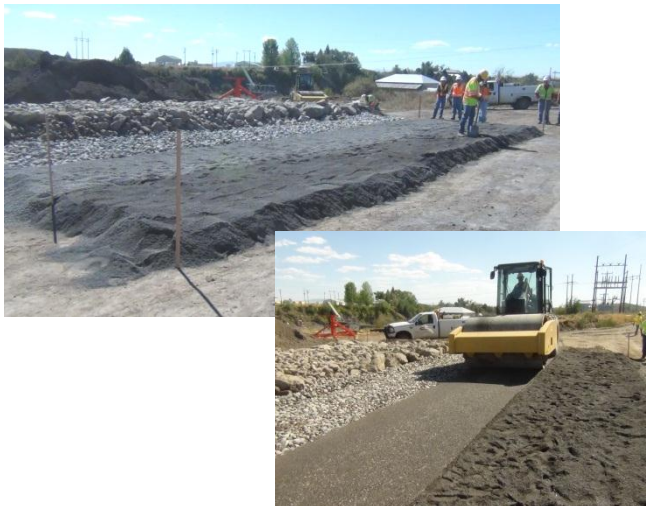
Photo 3. Test Pad for Granular Filter Materials
